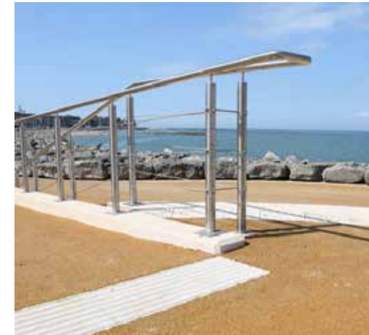
Porous coloured asphalt
