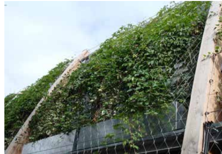
Green wall – trellis based system
