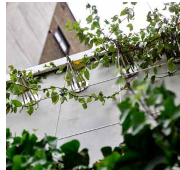
Green Wall - support structure
