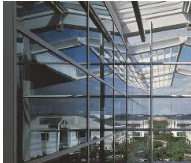
Cladding and solar shade detail
