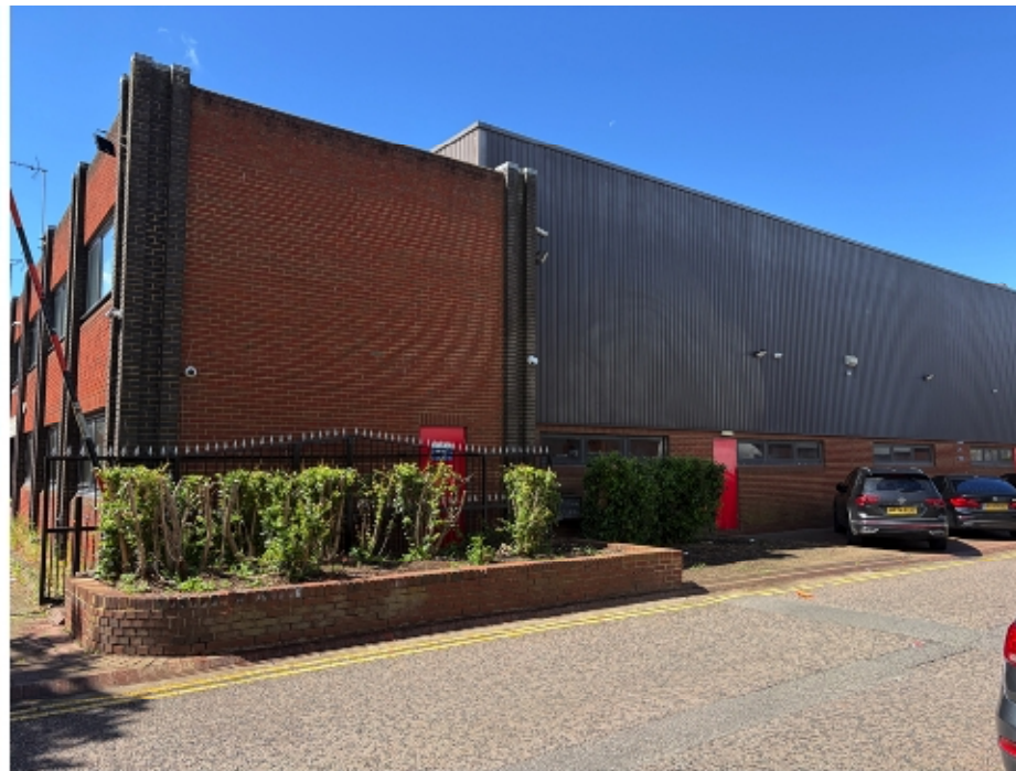
View of side of existing building along the access road
