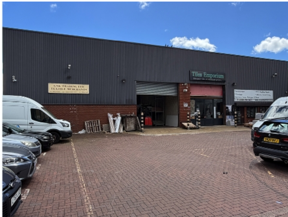
View of existing rear facade and service yard
