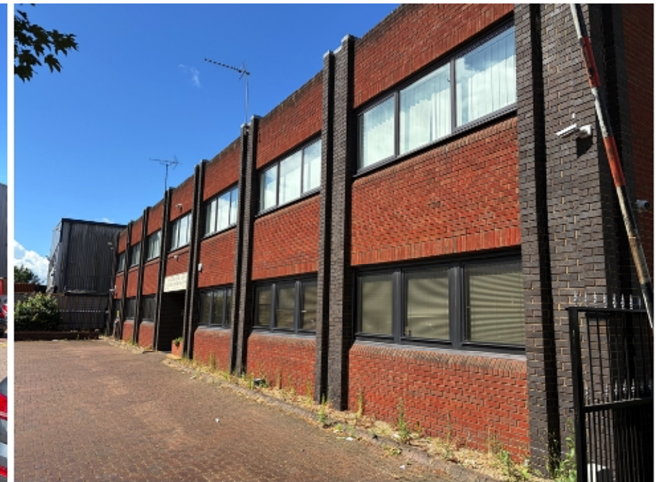
View of existing building frontage
