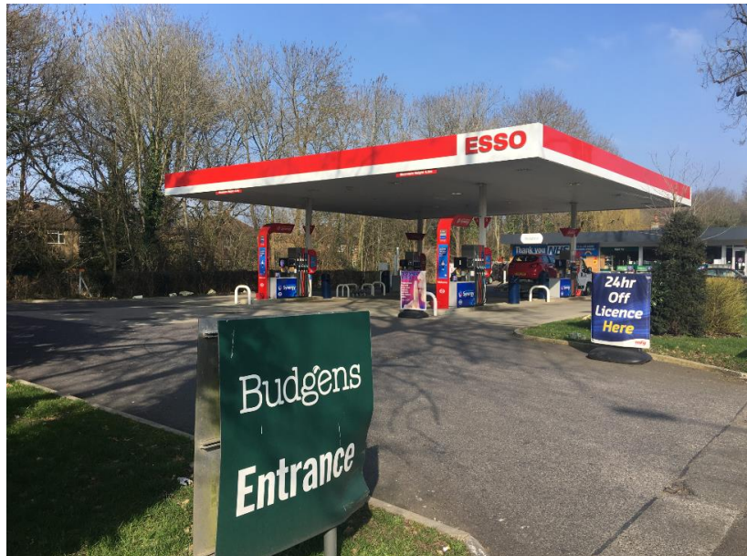
Pl.1: The service station from the High Road; note houses glimpses through trees to rear.
