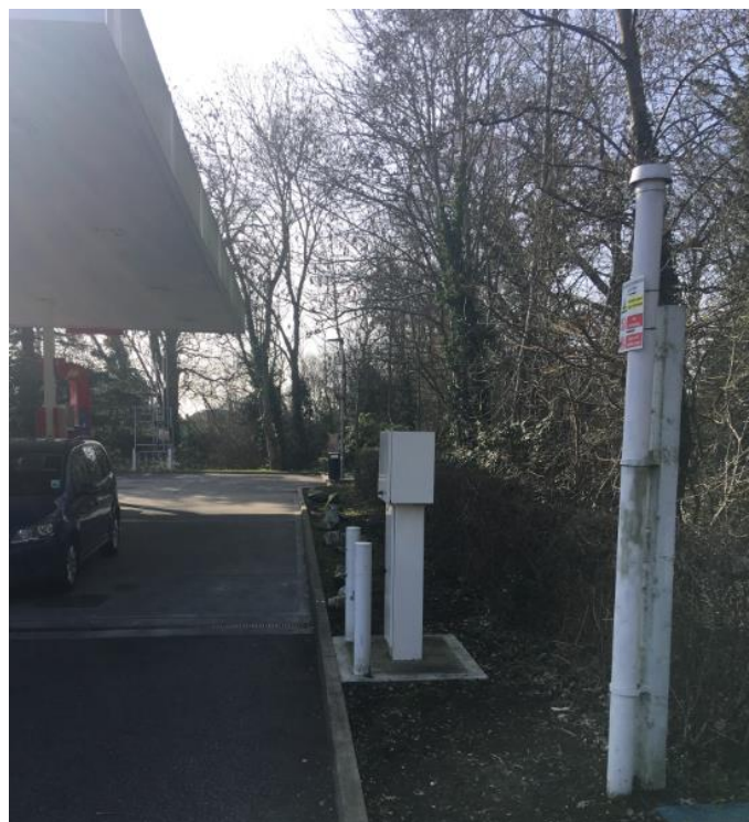
Pl.9: Existing garage paraphernalia along the rear boundary of the forecourt.
