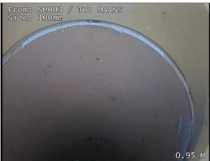
Line of drain/sewer deviates down
