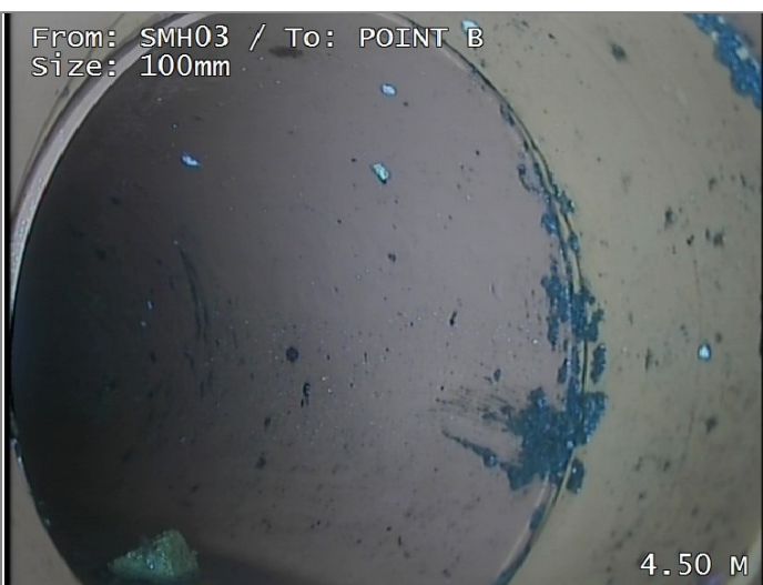
Line of drain/sewer deviates left
