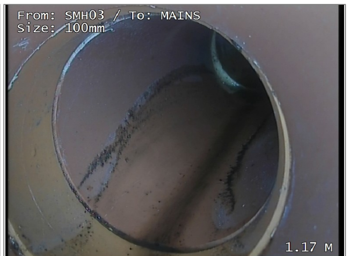
Line of drain/sewer deviates up
