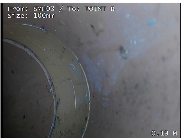
Line of drain/sewer deviates left
