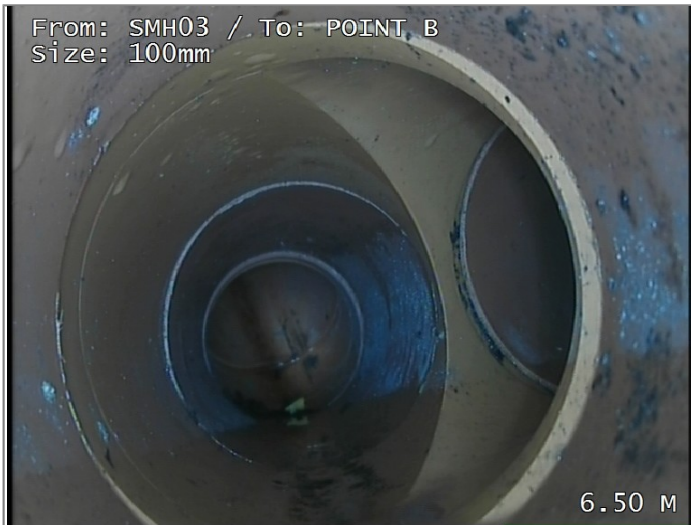
Junction at 3 o'clock, diameter 100mm - Remark: RDP06
