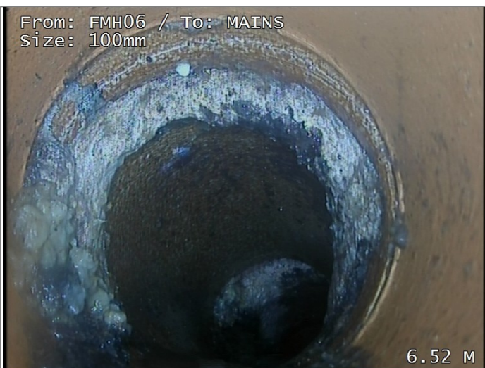
Attached deposits, encrustation from 12 to 12 o'clock 30% cross-sectional area loss
