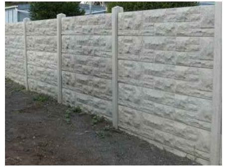
1 1.8m Conc. fence panels & conc. posts (CONDITION 4)
