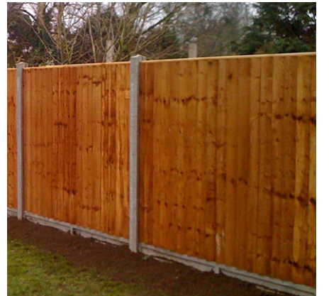
2 1.4m Timber fence panels & conc. posts (CONDITION 4)
