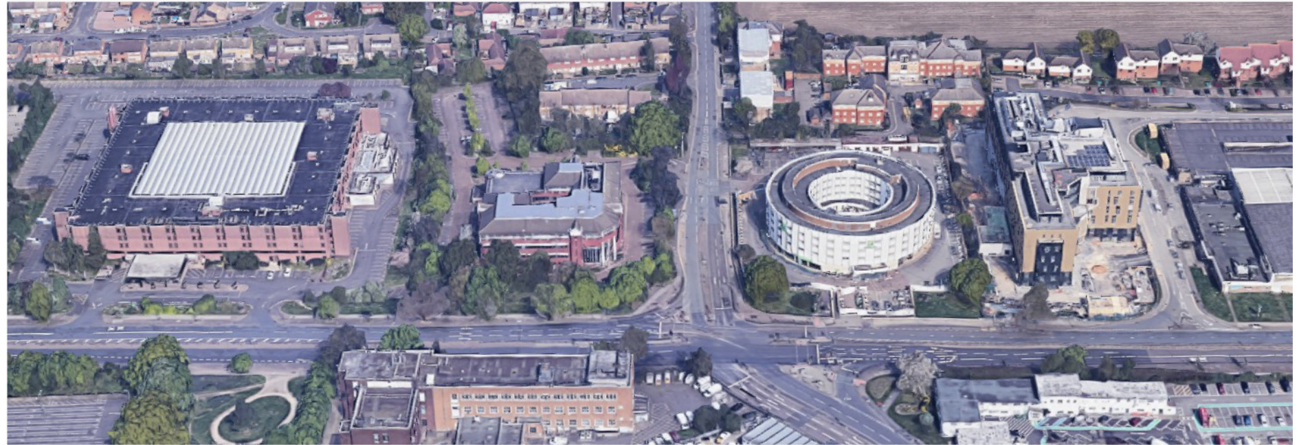
Aerial view looking north to the site showing the Bath Road frontage
