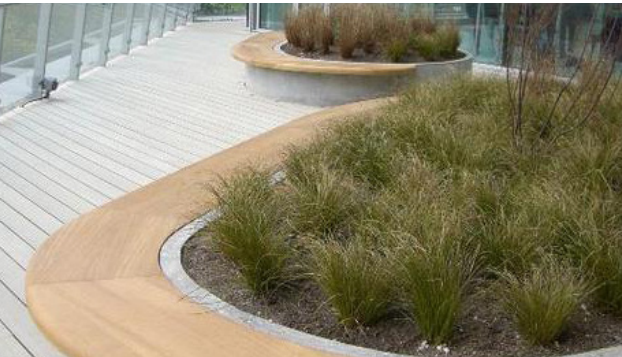
Curved timber seating to concrete upstand
