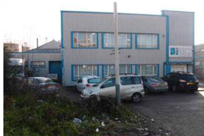
4 Existing light-industrial building at 3 Viveash Close
