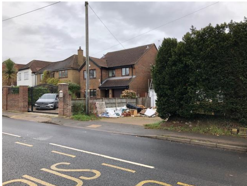
Pillars and gate at the application site lower than the hedging at 244 Northwood Road
