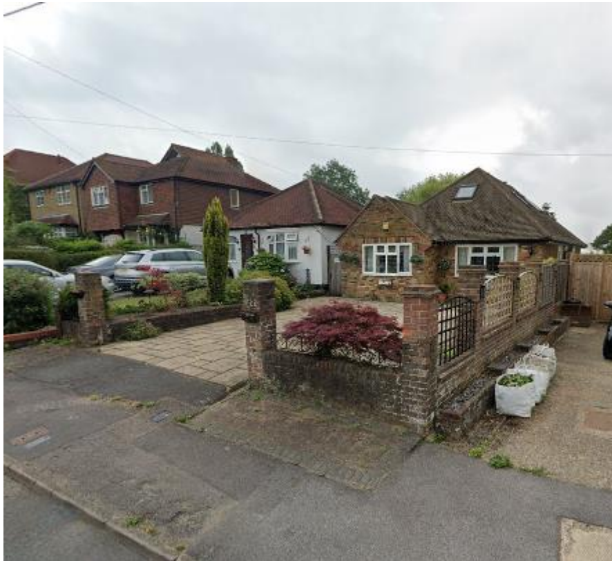
Walls, pillars, and railings
