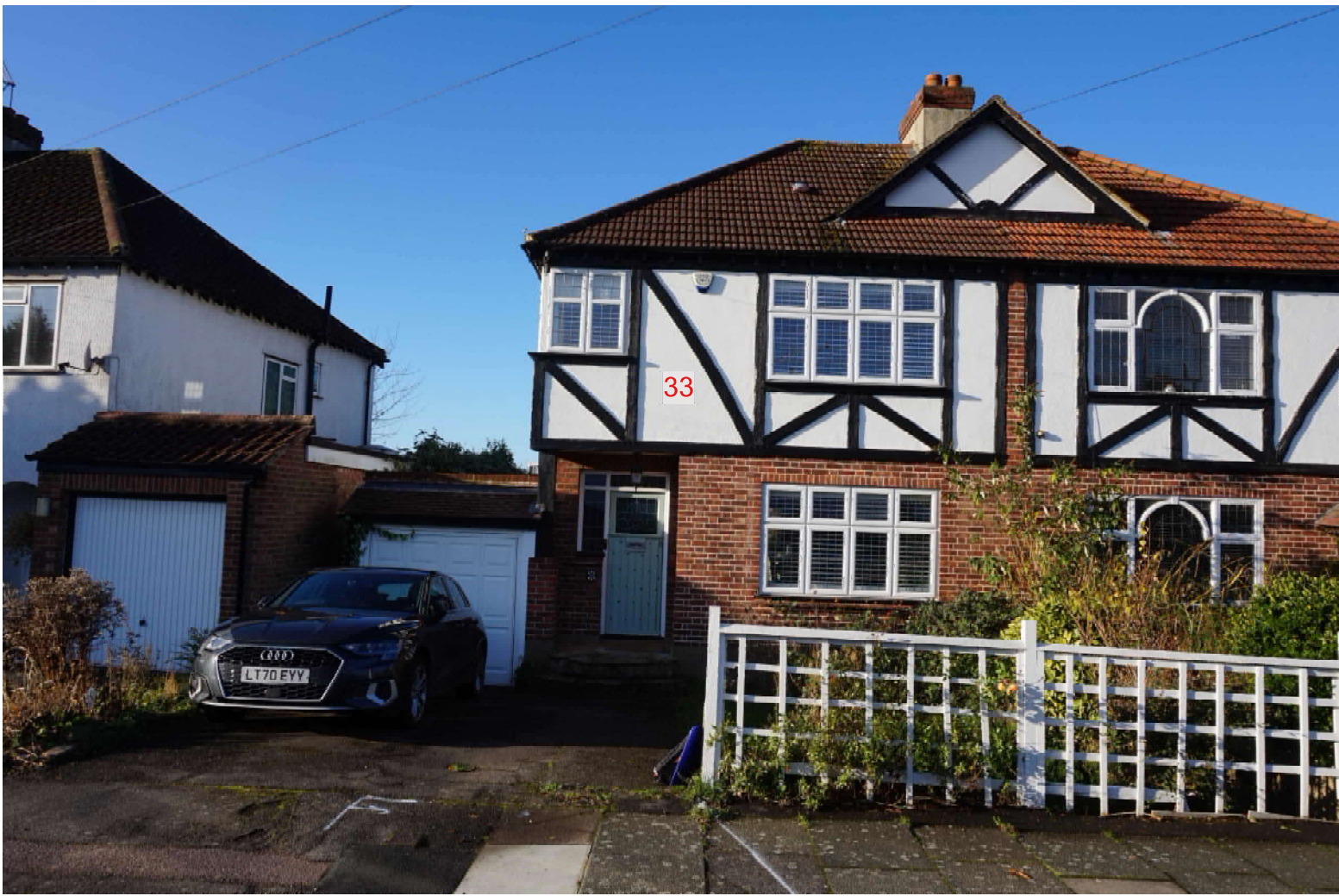
VIEW - FRONT (STREET)
