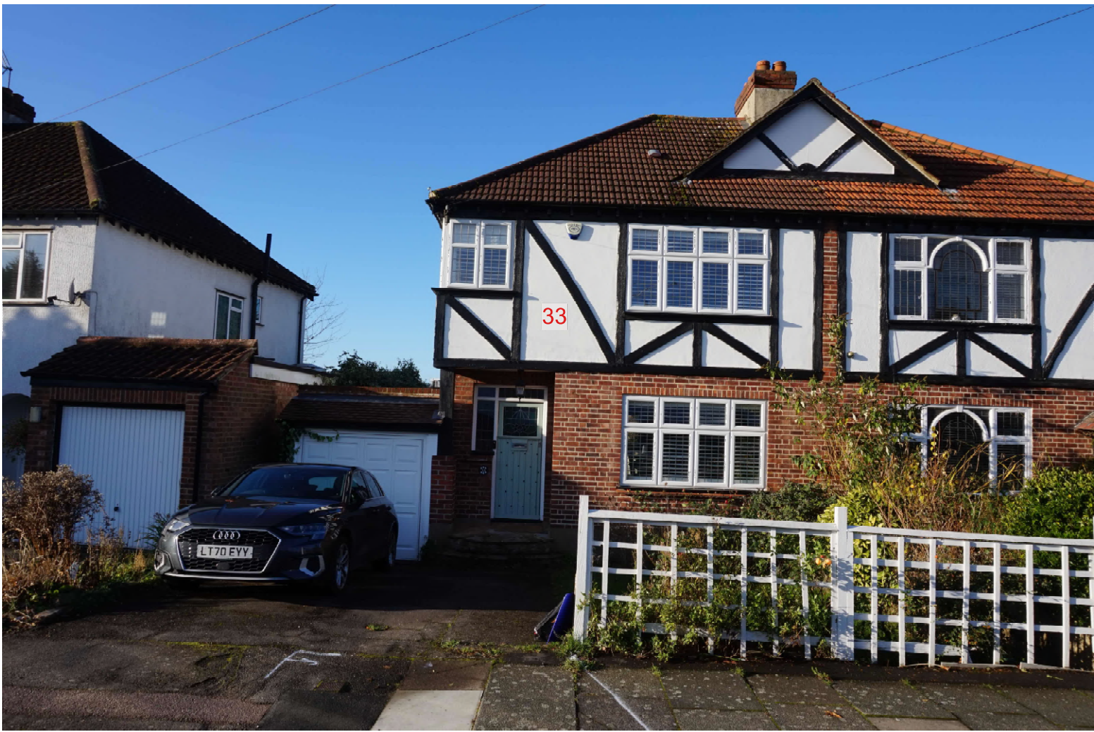
VIEW - FRONT (STREET)
