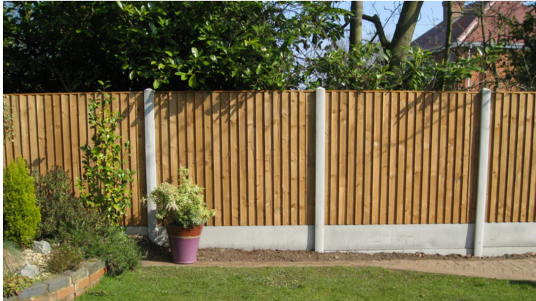
close-boarded timber fencing
