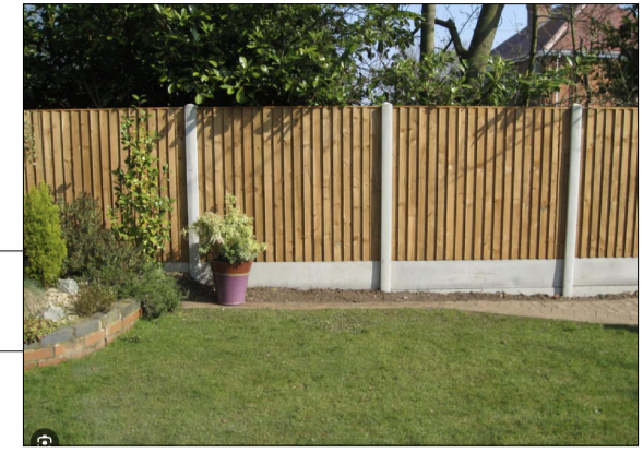
1.8m close-boarded timber fencing with gravel board and concrete posts.
