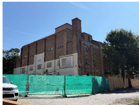
View facing B1 (rear of the property)
