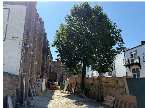
View facing down the southern boundary
