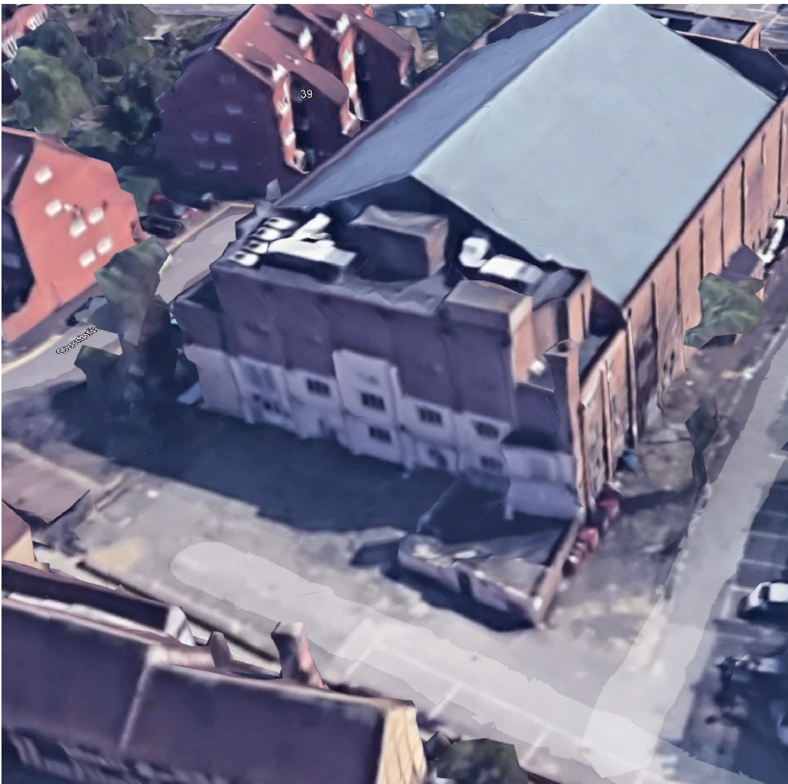
New extension on the rear of the existing building
