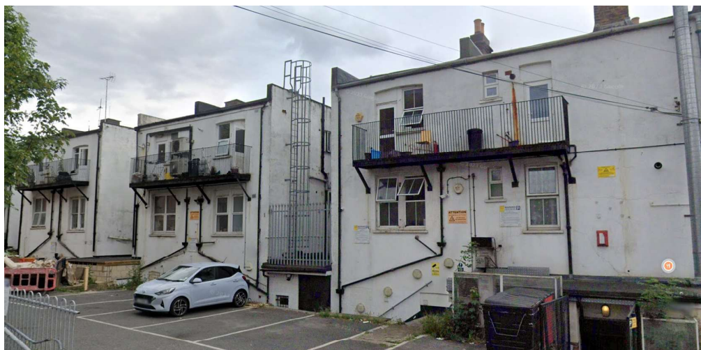
Fig 03 - 224 to 229 High Street (Source: Google Earth)
