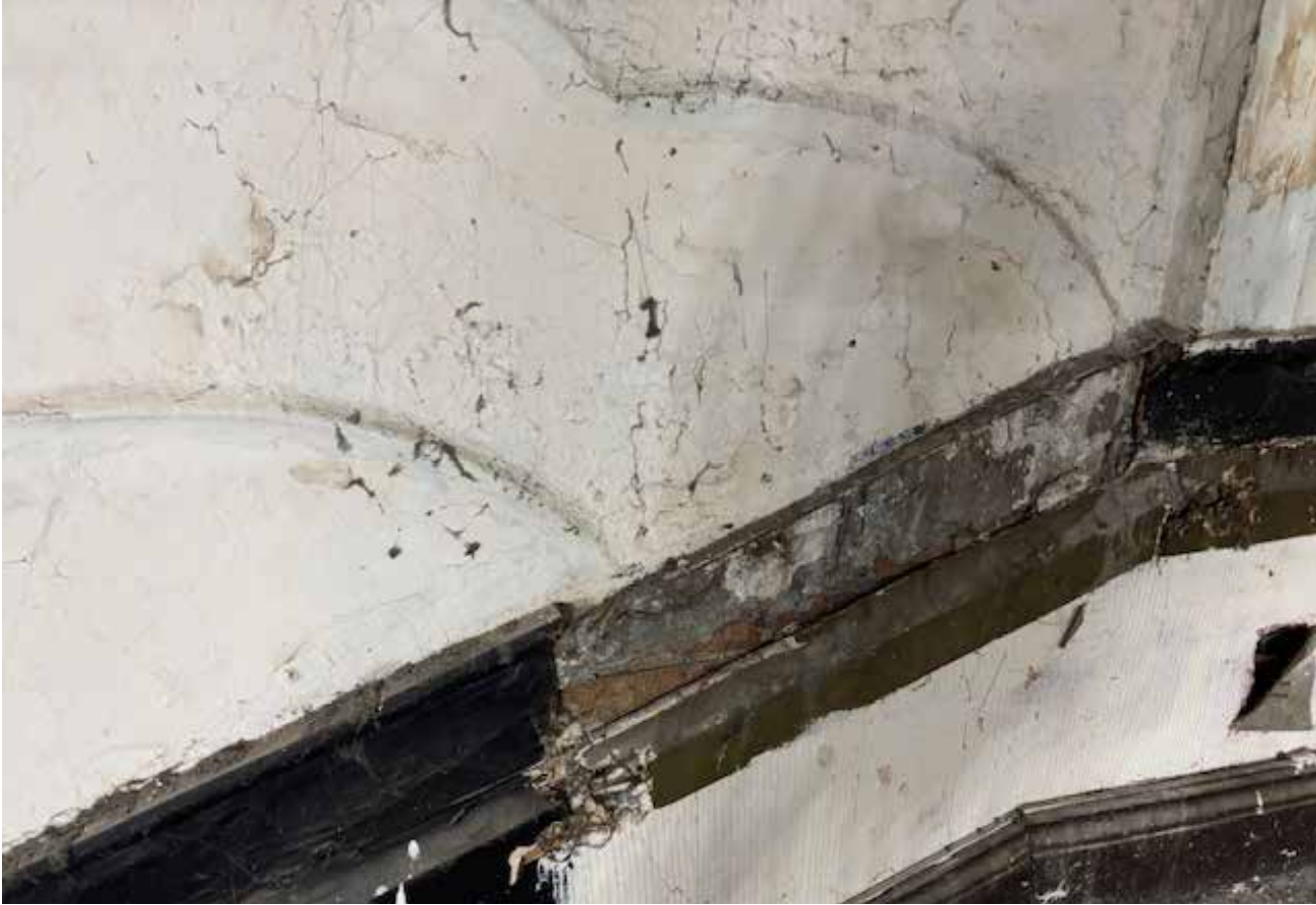
Damage to moulding and plaster revealed behind nightclub walls.
