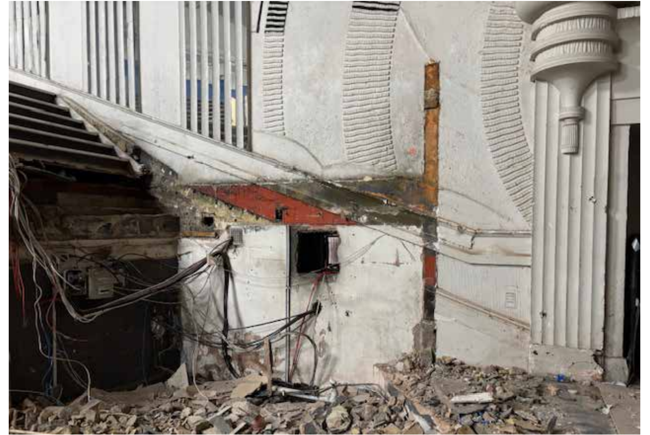
Mezzanine nightclub stairs removed and original plaster work exposed.
