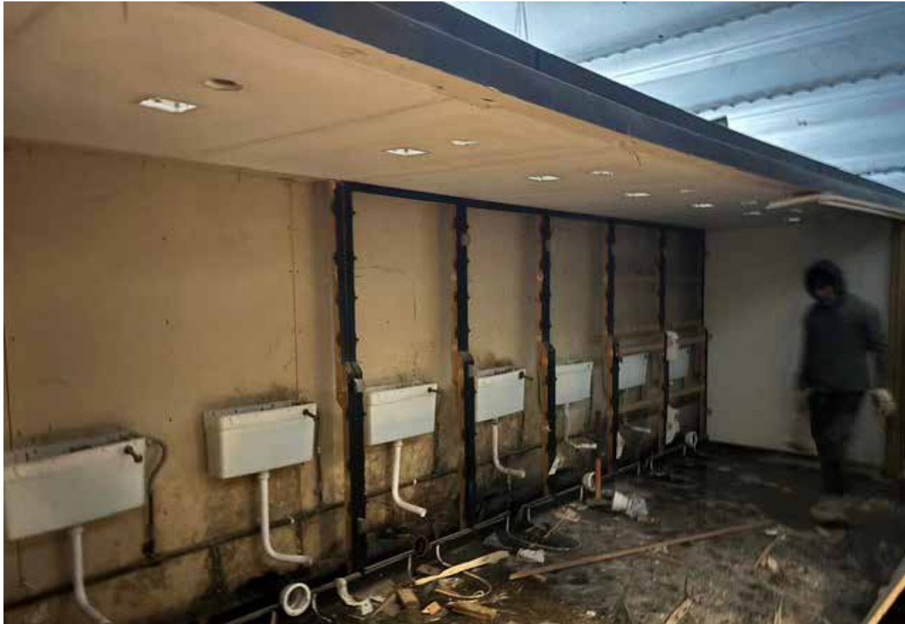
WC spaces carefully disconnected and removed.
