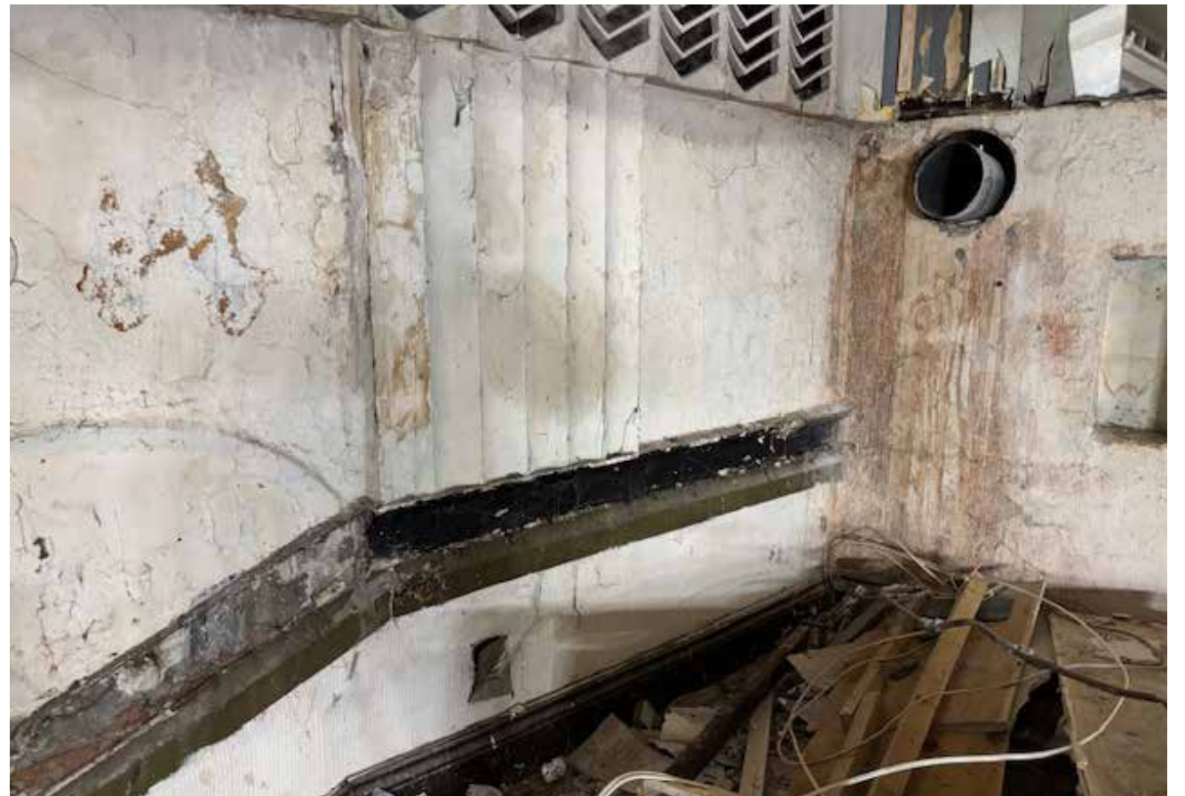
Original plaster work to upper side wall and damage caused prior to demolition of nightclub features.
