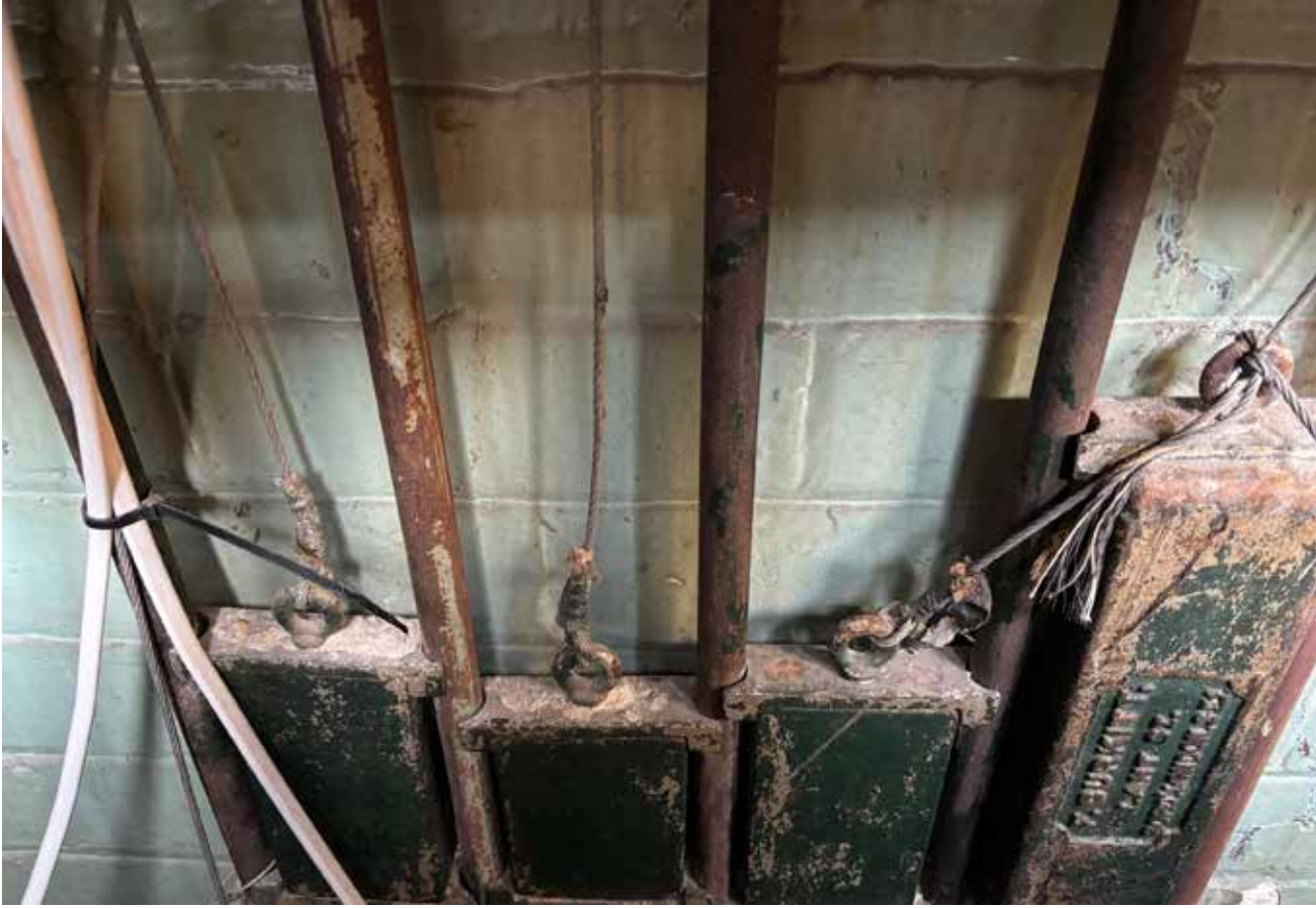
Original weight and pulley system revealed - possible smoke extraction vents.
