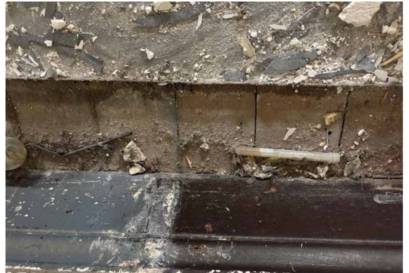
Original mezzanine timber floor exposed.
