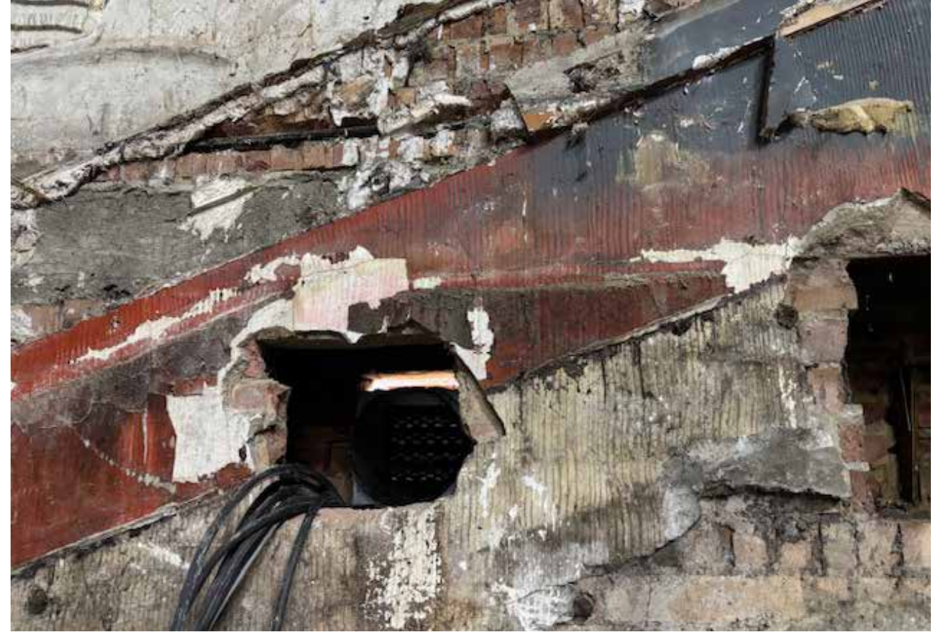
Damage to moulding and plaster revealed behind nightclub walls.
