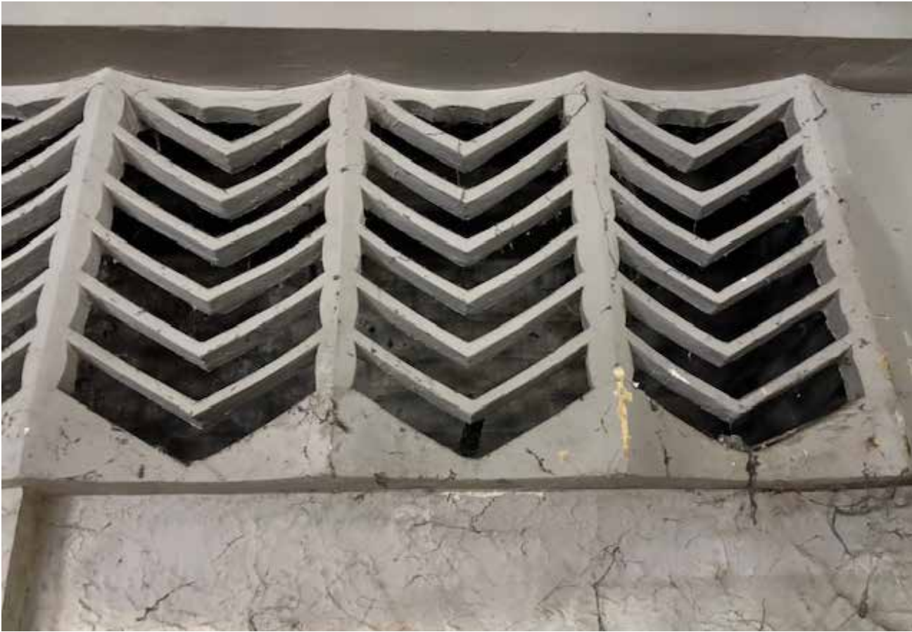
Original heating vents exposed in plaster work.
