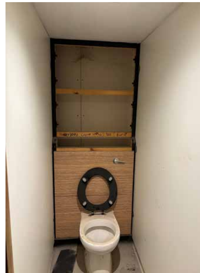
WC cubicles carefully demolished.
