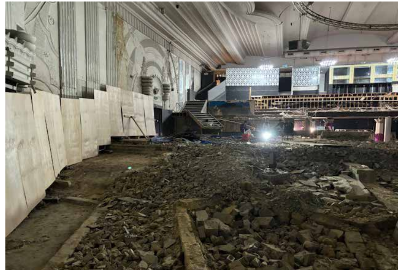
Auditorium floor debris removed and lower pit area debris removed.
