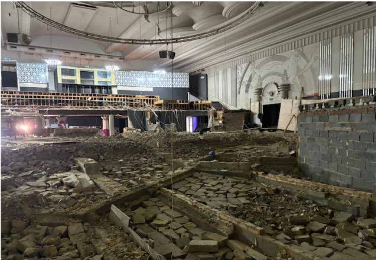
Auditorium floor debris removed and lower pit area debris removed.
