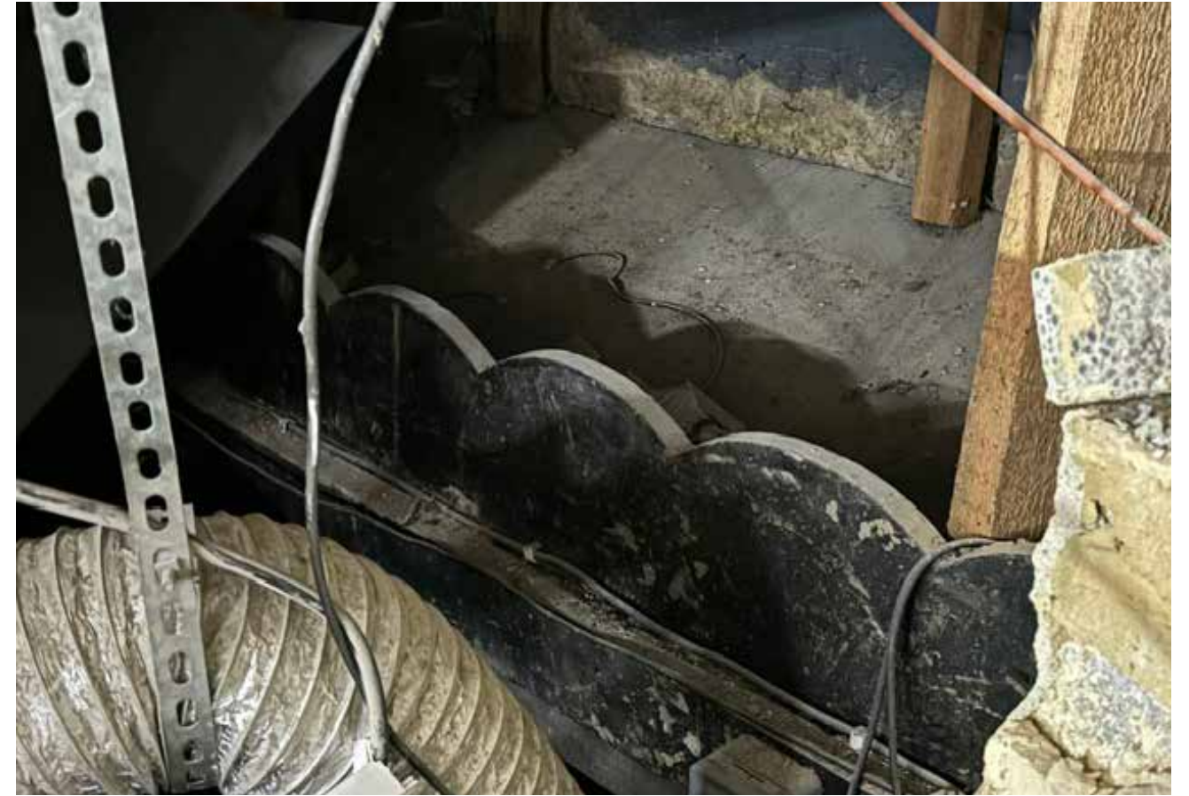
Original cinema stage edging exposed and retained.
