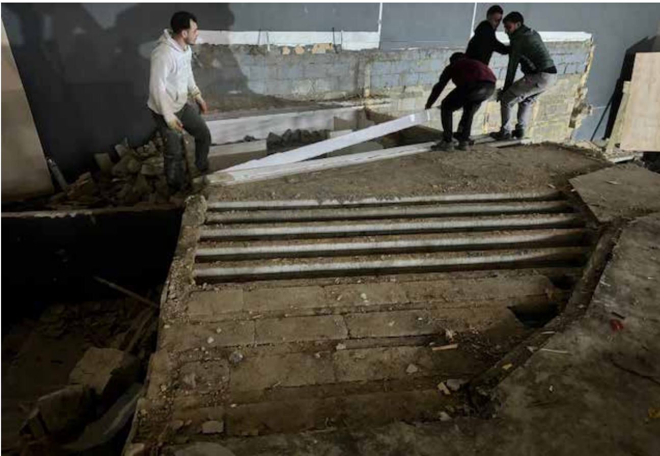
Original cinema stage edging exposed and retained.
