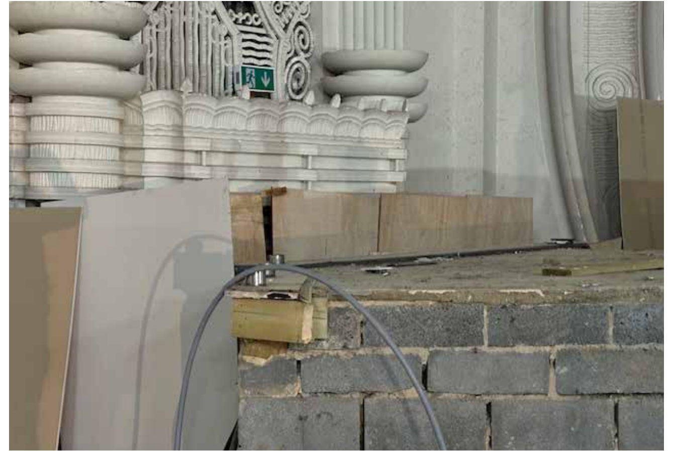
Original cinema stage edging exposed and retained.
