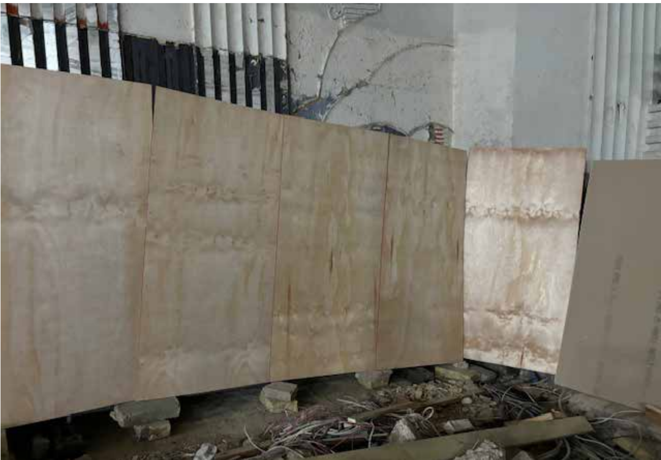
Plywood hoarding installed - 300mm away from listed plaster features.
