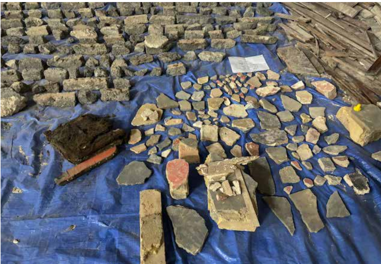
Original plaster and finishes collected and stored.
