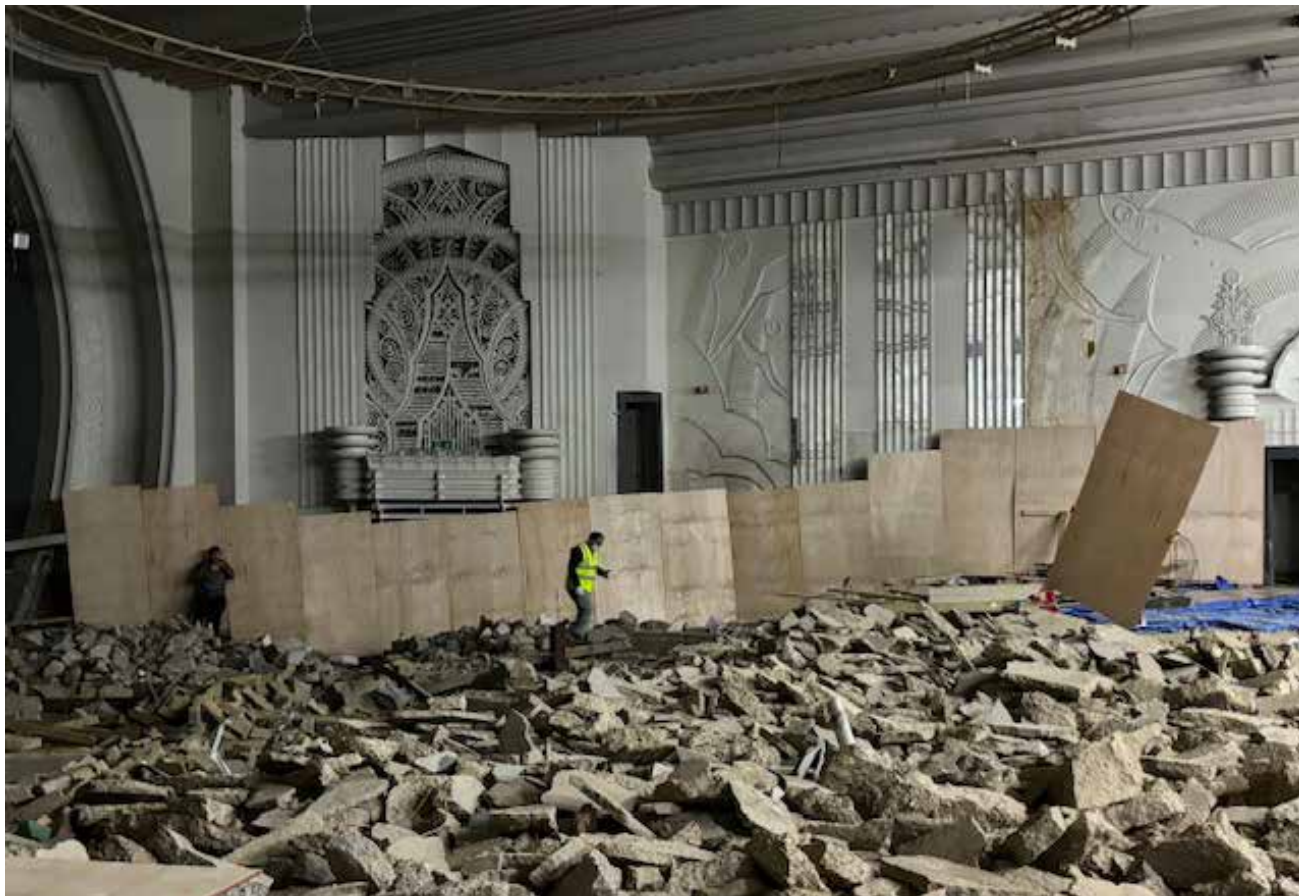
Auditorium floor debris and hoarding being installed.
