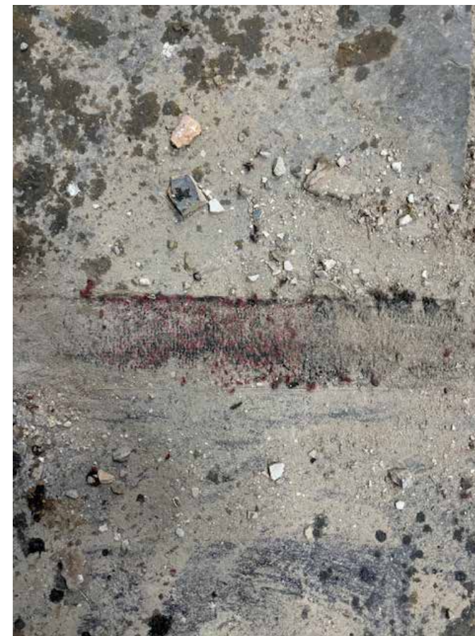
Carpet strip in floor - potentially original cinema floor.
