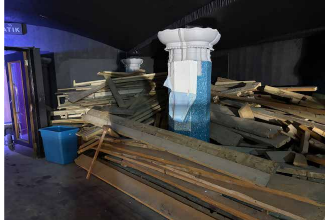
Timber floor structure from the nightclub mezzanine ready for removal.
