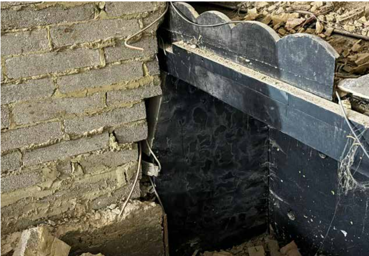
Original cinema stage edging exposed and retained.
