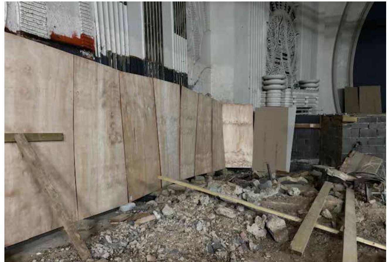
Hoarding installed and auditorium floor rubble ready for removal.
