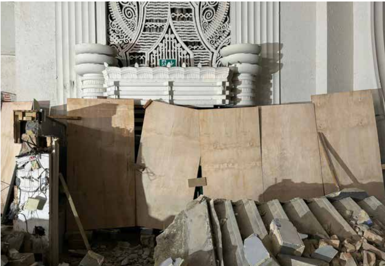
Lower entrance area protected during demolition of the modern bar enclosure.
