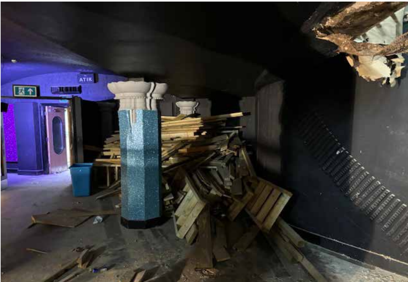
Timber floor structure from the nightclub mezzanine ready for removal.
