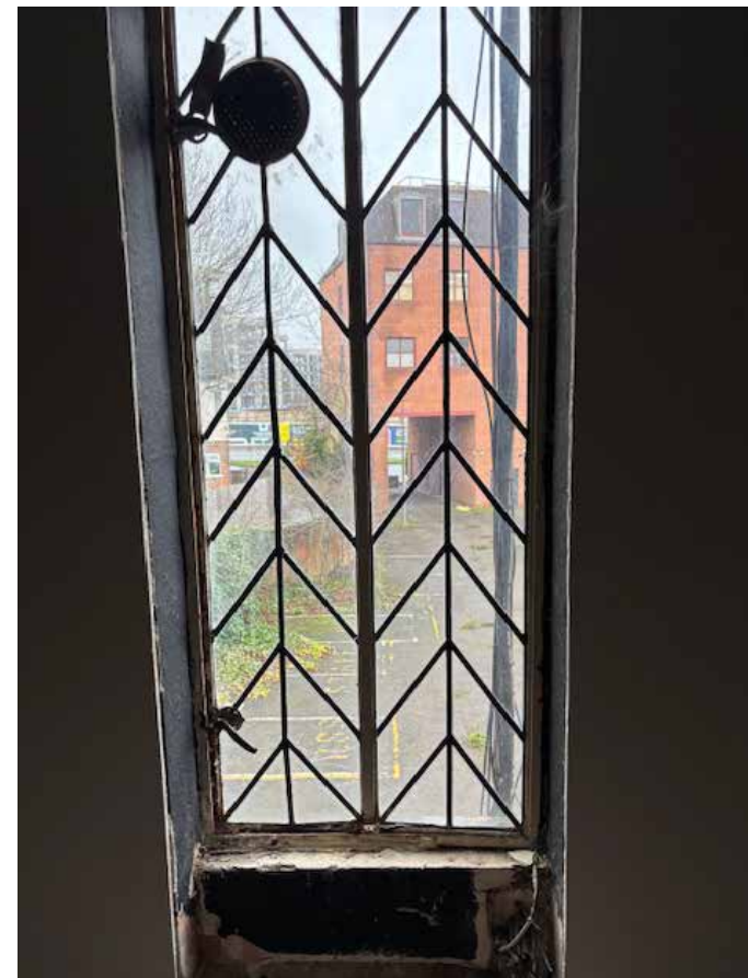
Original lead work to windows.
