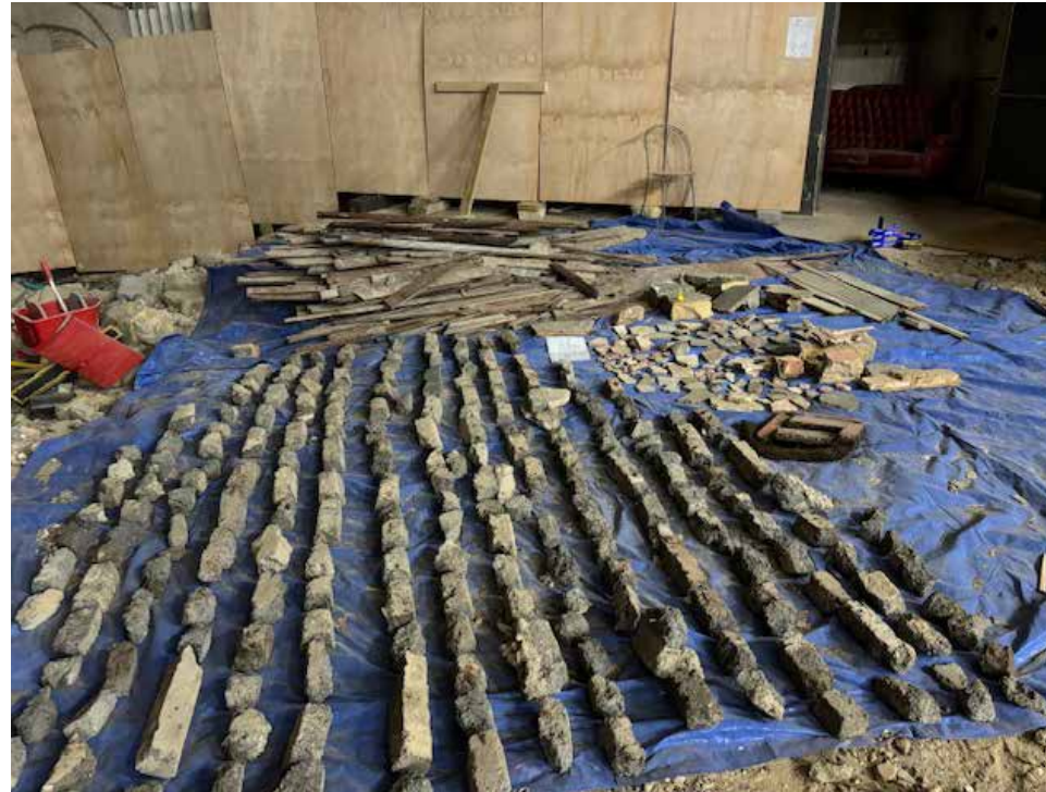
Original clinker floor blocks that supported the original timber floor.
