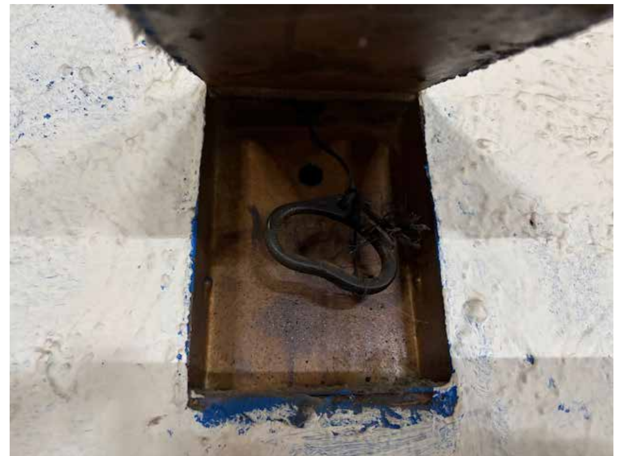
Original pull handle for cinematographer hatches.
