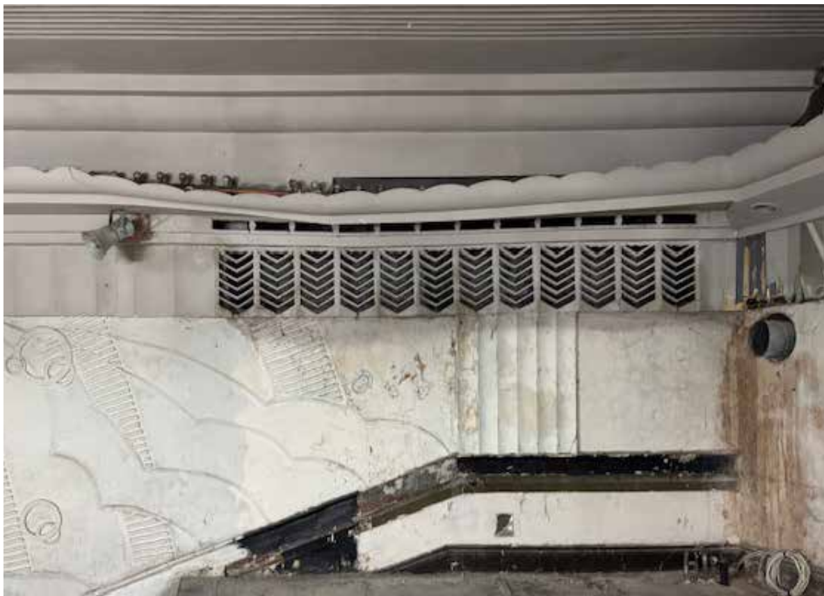
Original plaster vents to the upper floors.
