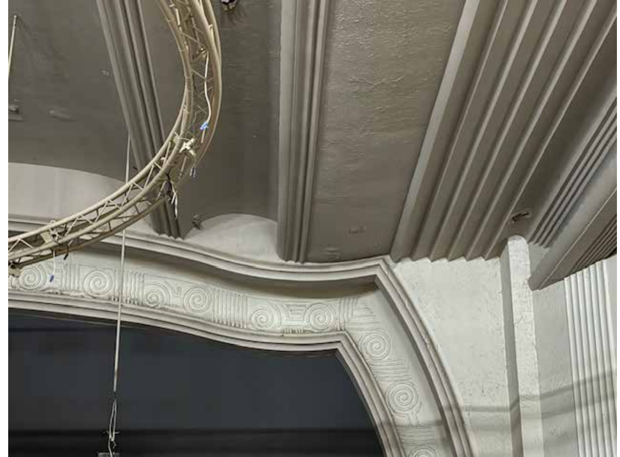
Original wall, ceiling plaster work retained. Small areas of water ingress damage.
