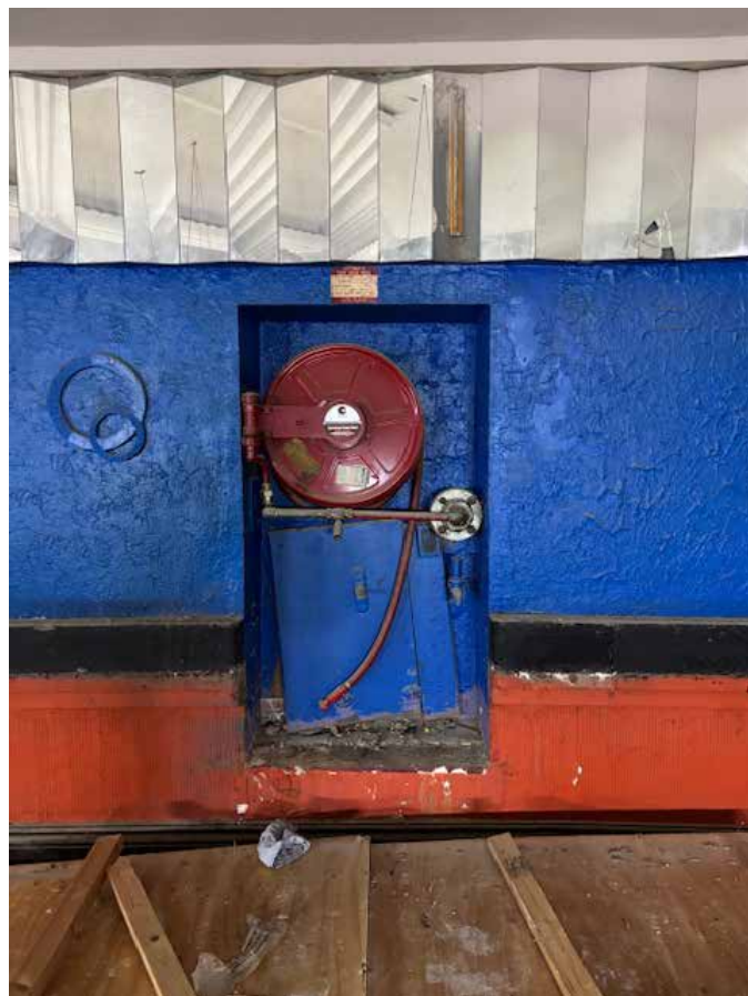
Original plaster detailing and hydrant alcove.
