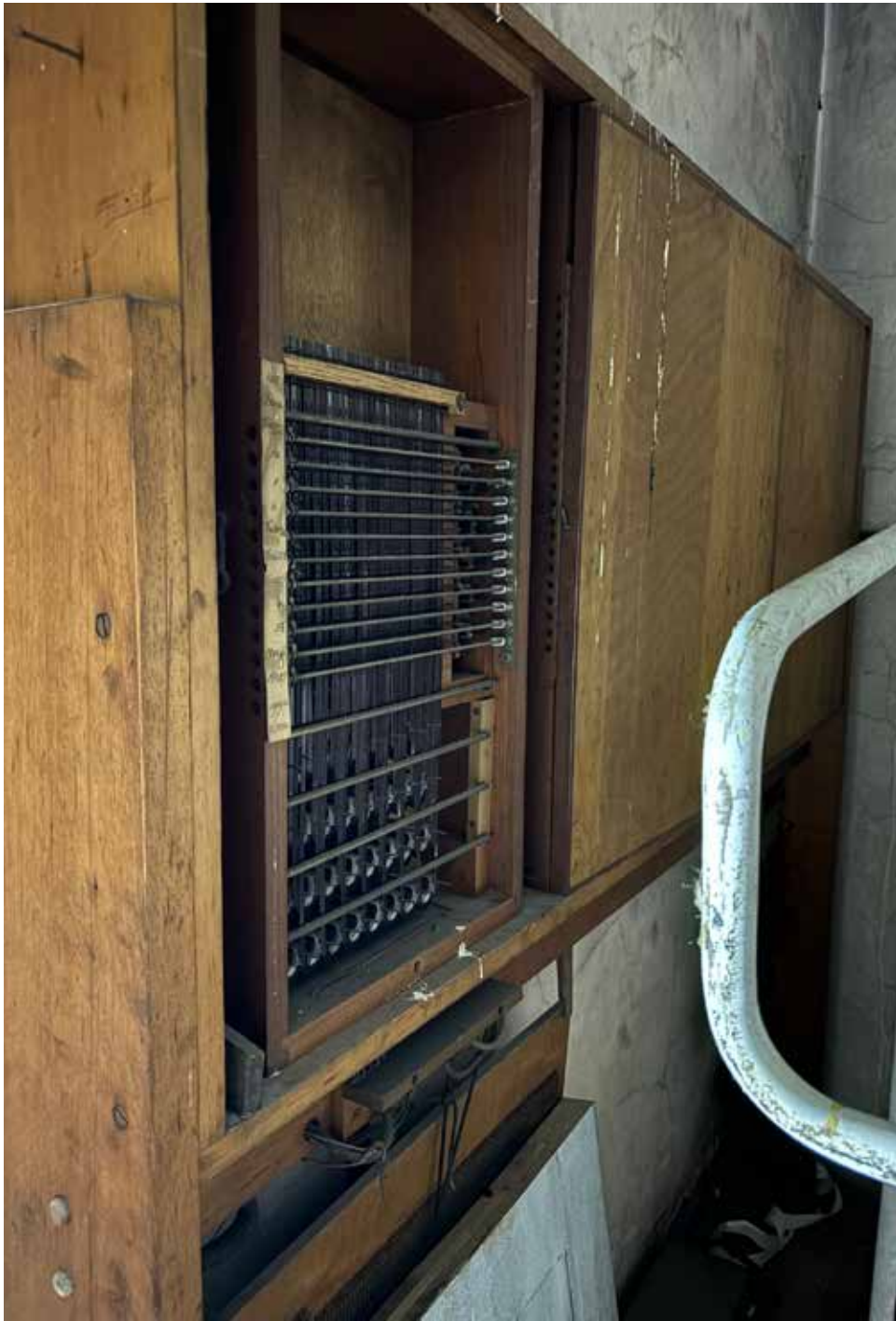
Musical and lighting equipment in original enclosures and cabinets. The referred to “Western Electric system of sound apparatus”
