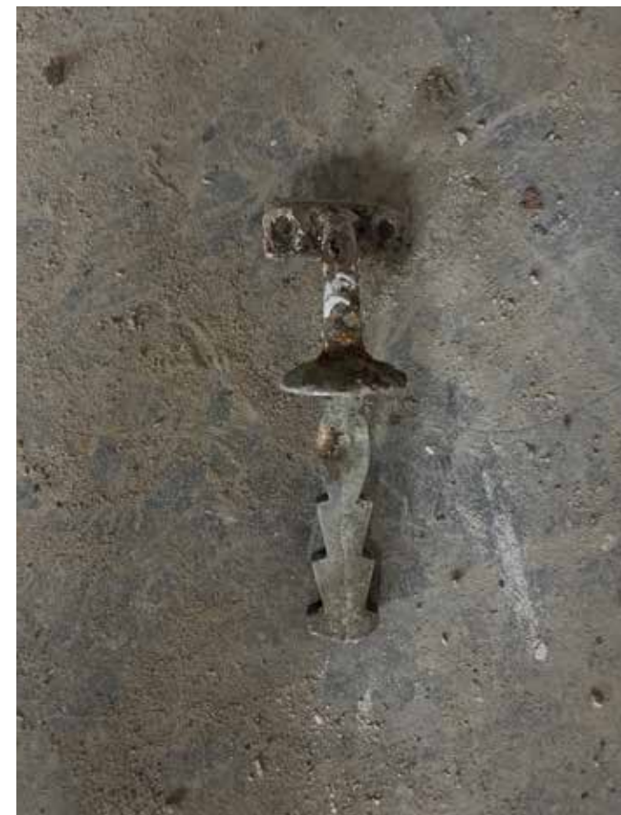
Original metal connection for the cinema handrail.
