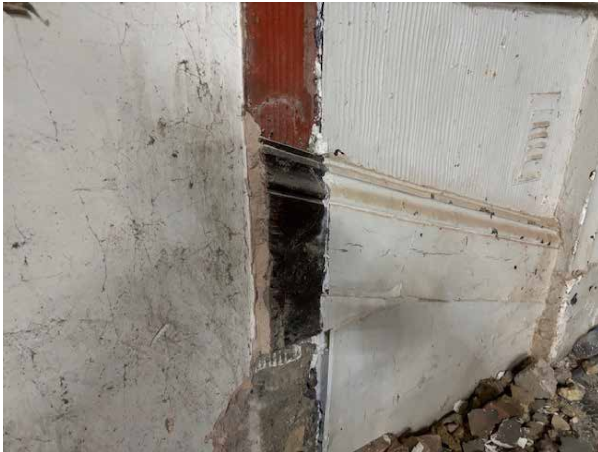
Original sloped dado and painted timber work.
