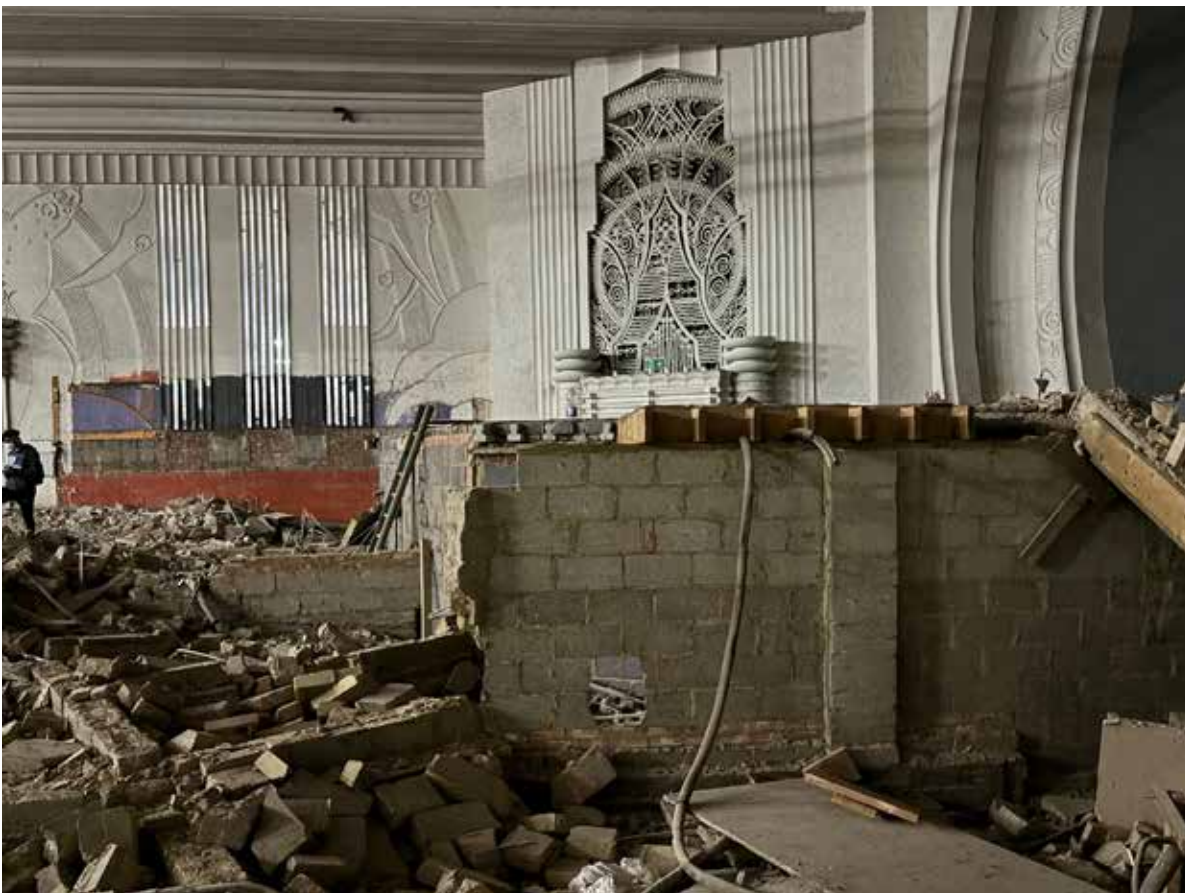
Exposed and part demolished block walls to form a stage in the night club use.
