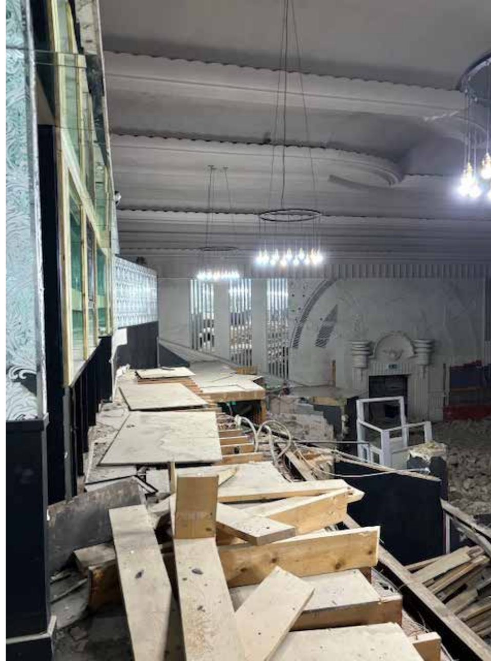
Night club mezzanine partly removed. Wall cladding to the left sits in front of the original plaster work.
