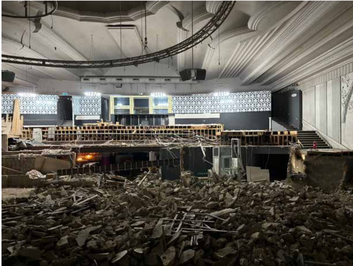
Night club raised floor demolition, with night club mezzanine partly removed in the background.
