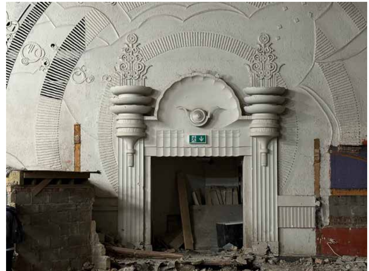
Cinema exit door detailing, plaster work still intact. Damage to walls have been caused by the raised night club floor.
