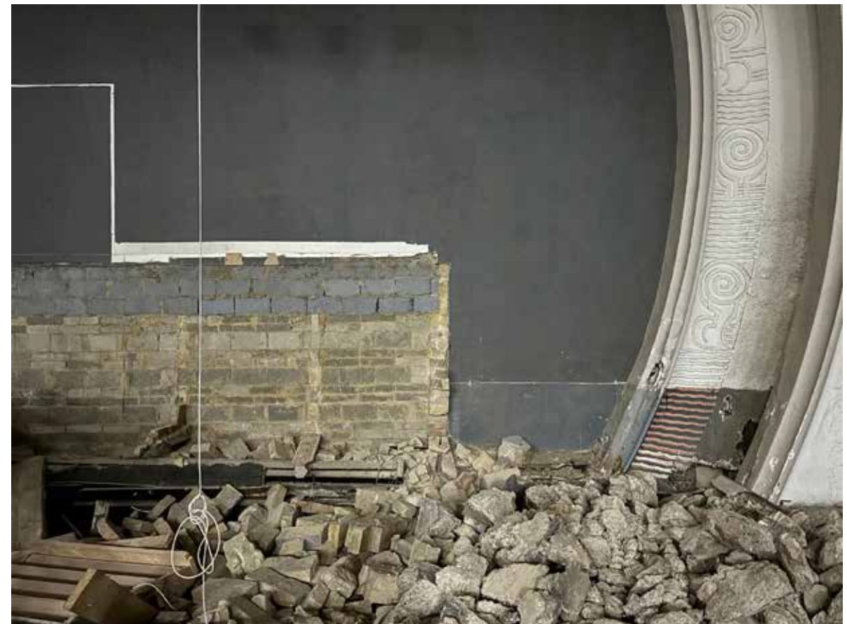
Night club podium and raised floor demolished, rear wall plaster work intact.
