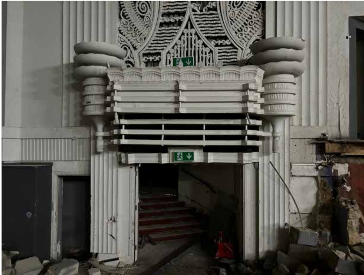
Plaster work and fluting around exit doors. Damage to wall as a result of nightclub floors
