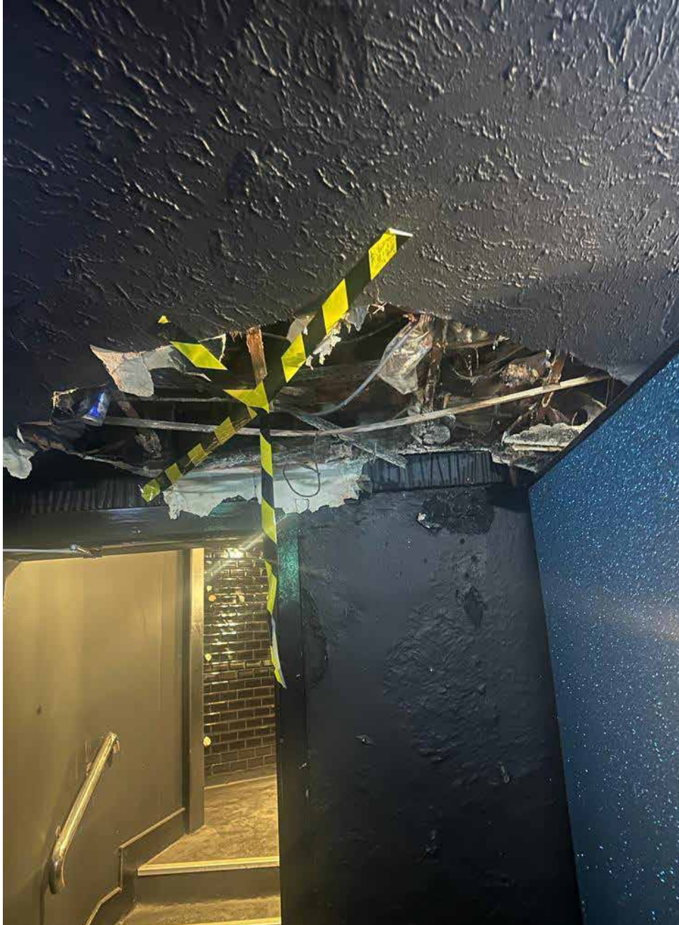
Water damage to the plaster work from roof leaks.
