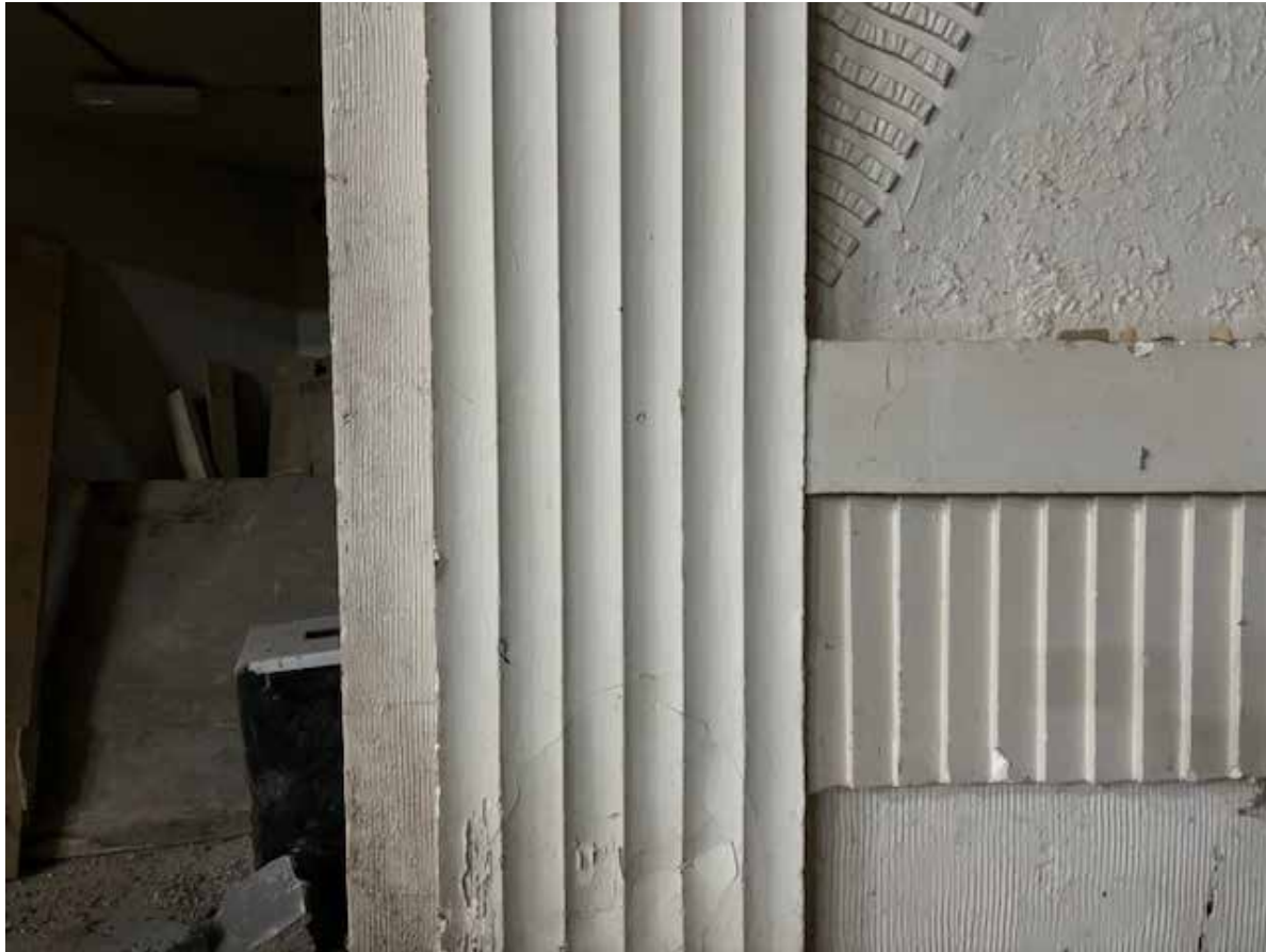
Original plaster wall panels retained with areas of damage following the night club floor levels.
