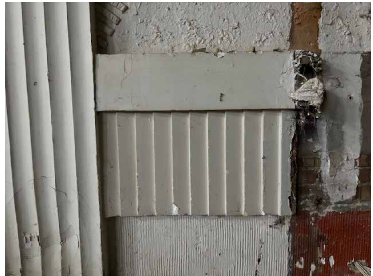
Original plaster wall panelling with areas of damage caused by previous night club floor structures.
