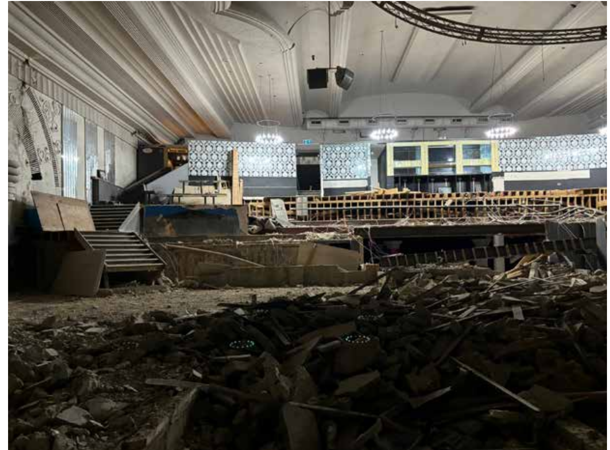
Raised night club floor demolished, Night club mezzanine removed partially.
