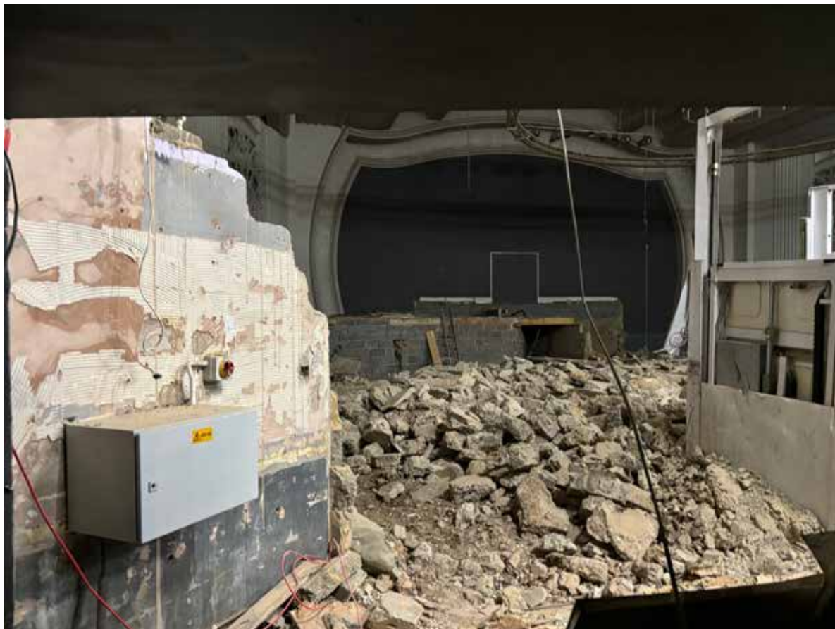
Nightclub floor and stud walls demolition. Cinema wall and panelling retained.
