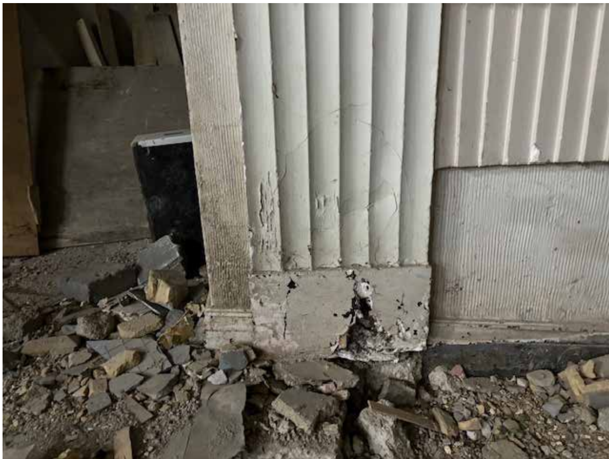
Original plaster wall fluting and panelling with areas of damage at floor level.
