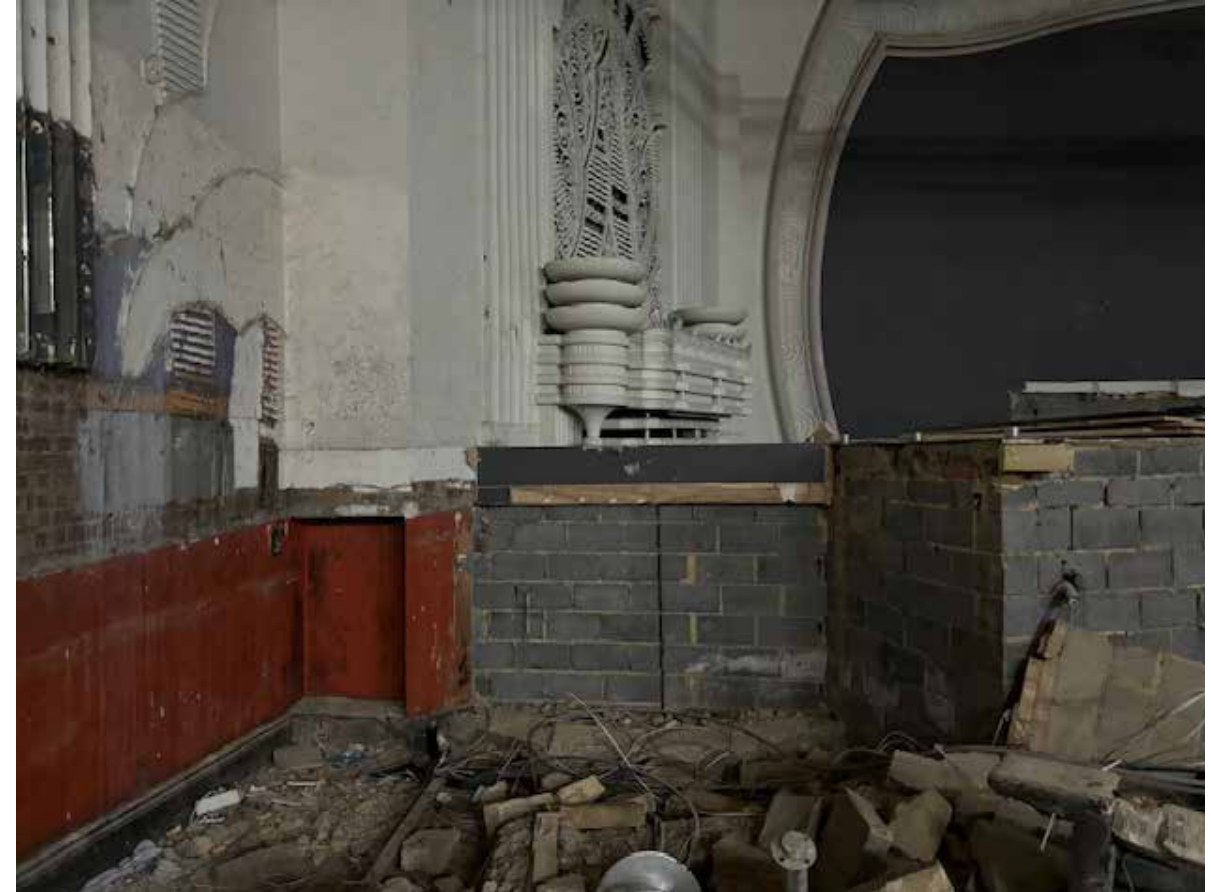
Current condition of the cinema space, block work walls to later night club alterations.
