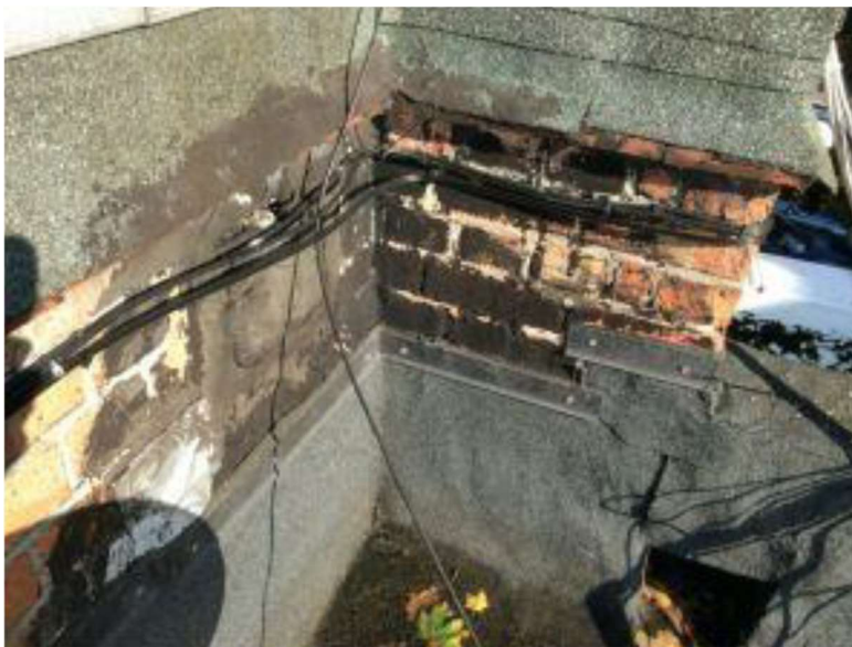
Img 6 Bituminous liquid patch repairs to brick upstands on main roof area. Despite mineral felt termination bar detail there are still ongoing moisture ingress problems. Note electrical cabling fixed to parapet wall.
