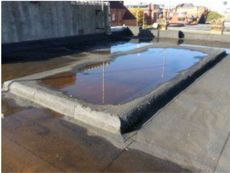
Img 3 Standing water on decked over rooflight aperture to main roof area.
