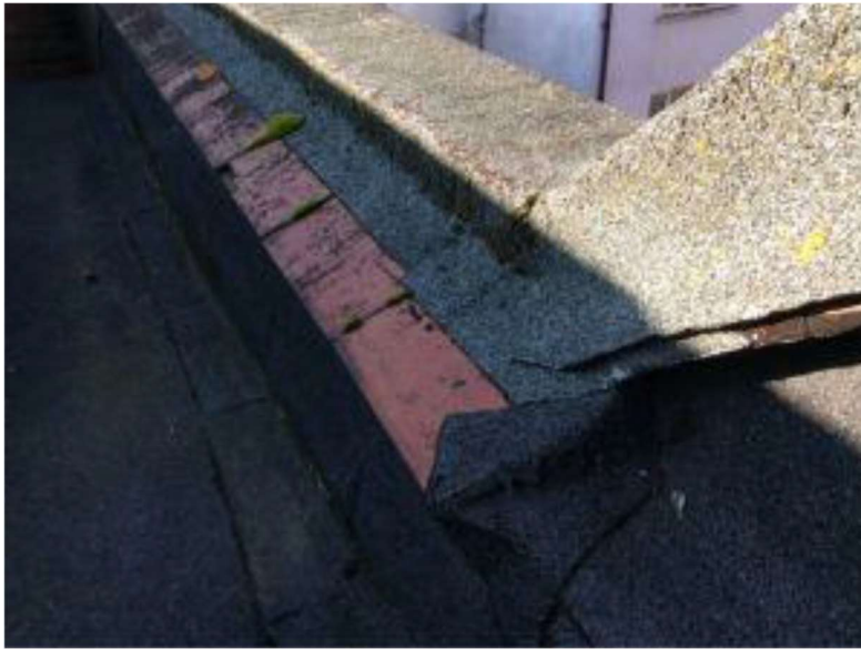
Img 7 Parapet walls have been partially encapsulated with felt to the inner leaf and top without terminations.
