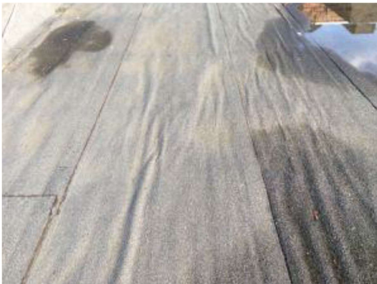
Img 4 Rucking due to trapped moisture vapour to main roof area.
