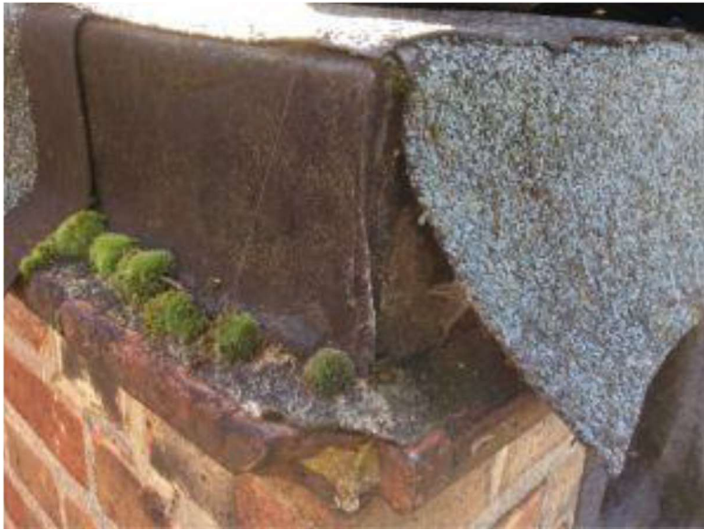
Img 5 Poor termination of waterproofing to outer of edge of parapet wall. Note: organic growth indicating areas of standing water.
