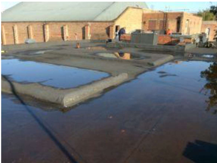
Img 2 Main roof area overview as above showing severe ponding indicating poor falls and place additional load the roof area as well as presenting a severe slip hazard if maintenance is required in ice cold weather conditions.
