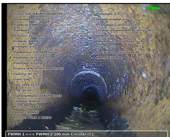
20190615-105947-snap0000.jpg, 00:00:01, 0.00 m Start node type, manhole, reference number: 1
