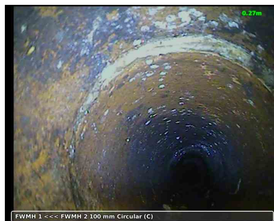
20190615-105947-snap0001.jpg, 00:00:21, 0.27 m Joint displaced, medium
