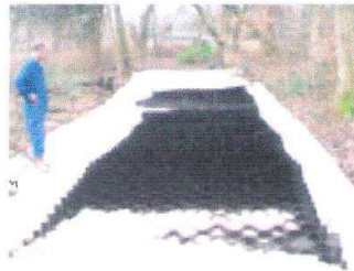
Installation of the CellWeb™ system.
