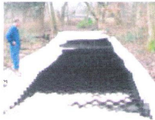
Installation of the CellWeb™ system.
