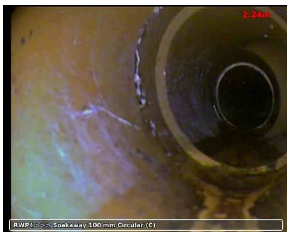
20210517-112820-snap0002.jpg, 00:00:46, 2.24 m Junction, at 03 o'clock, diameter: 100 mm
