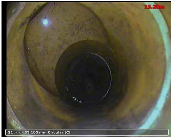
20210517-111415-snap0004.jpg, 00:01:25, 15.28 m Junction, at 09 o'clock, diameter: 100 mm
