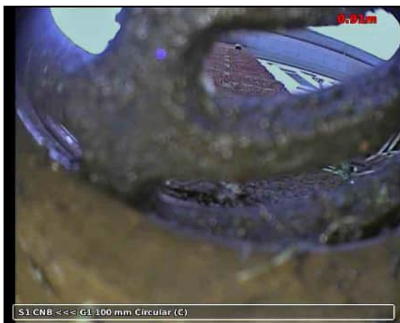
20210517-111300-snap0002.jpg, 00:00:40, 0.91 m Finish node type, major connection without manhole, reference number: G1
