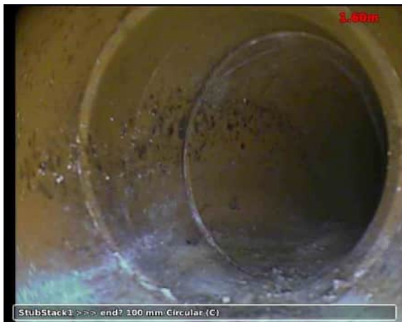
20210517-113048-snap0000.jpg, 00:00:31, 1.60 m Line deviates right
