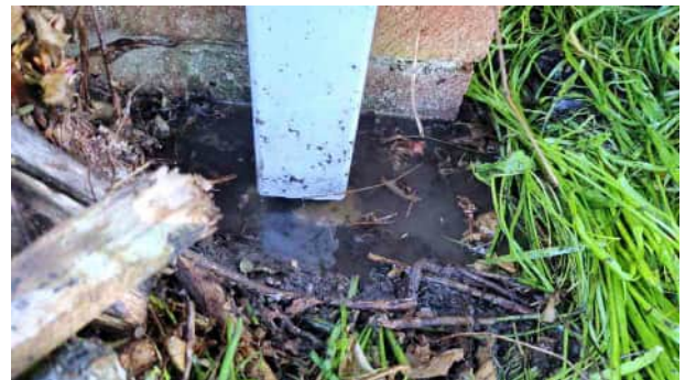
RWP1 - Discharges into ground. Not connected to below ground drainage.
