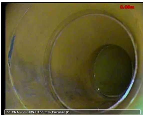
20210517-111107-snap0000.jpg, 00:00:16, 0.08 m Line deviates right
