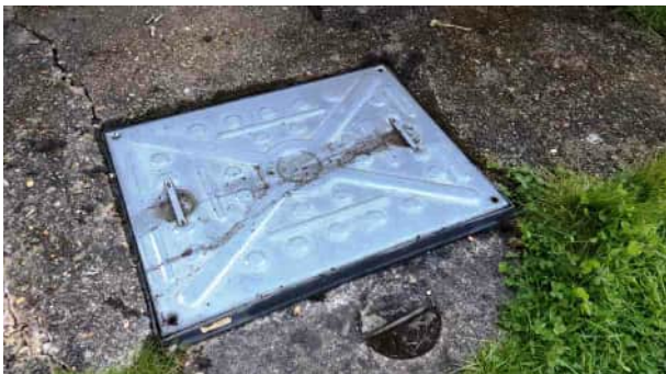
S1 - Manhole cover and frame is loose.
