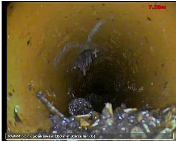
20210517-112820-snap0004.jpg, 00:01:08, 7.18 m Hole in drain or sewer, at 10 o'clock
