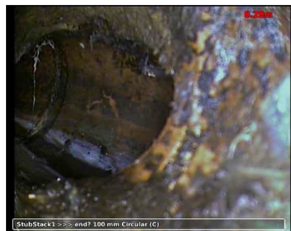
20210517-113048-snap0003.jpg, 00:01:35, 8.28 m Finish node type, major connection without manhole, reference number: Main Run
