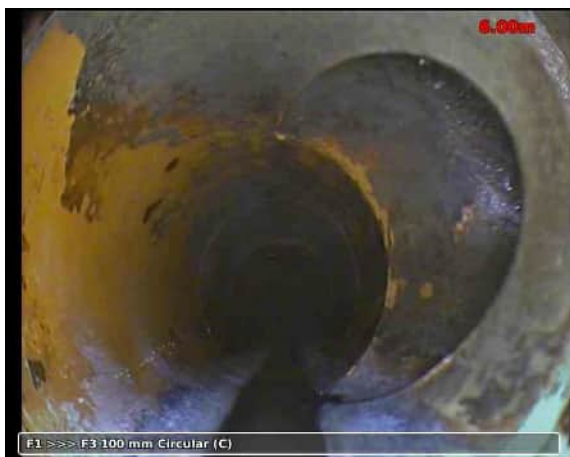
20210517-114655-snap0002.jpg, 00:00:25, 6.00 m Junction, at 03 o'clock, diameter: 100 mm
