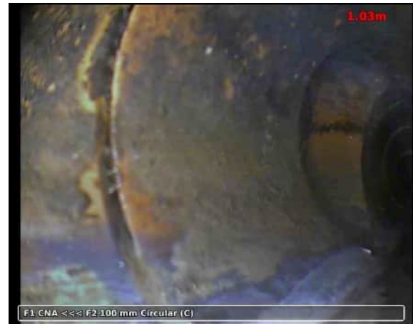
20210517-114036-snap0001.jpg, 00:00:36, 1.03 m Junction, at 09 o'clock, diameter: 100 mm
