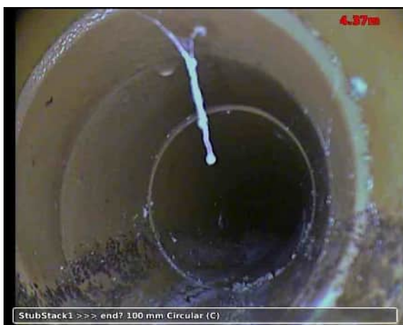
20210517-113048-snap0002.jpg, 00:00:45, 4.37 m Line deviates right
