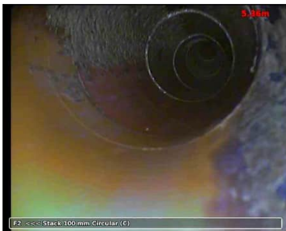
20210517-114529-snap0002.jpg, 00:00:39, 5.36 m Finish node type, major connection without manhole, reference number: Stack
