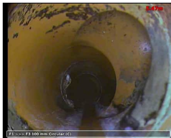
20210517-114655-snap0001.jpg, 00:00:19, 5.47 m Junction, at 03 o'clock, diameter: 100 mm
