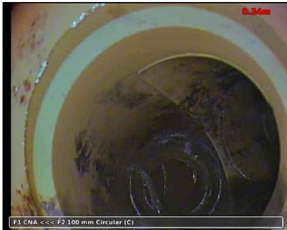
20210517-114036-snap0000.jpg, 00:00:14, 0.34 m Junction, at 03 o'clock, diameter: 100 mm
