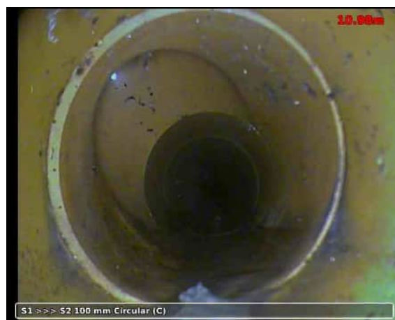
20210517-111415-snap0003.jpg, 00:01:07, 10.98 m Junction, at 09 o'clock, diameter: 100 mm
