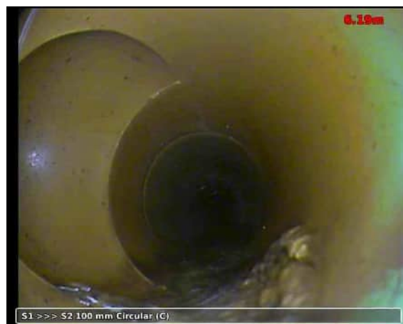
20210517-111415-snap0001.jpg, 00:00:26, 6.16 m Junction, at 09 o'clock, diameter: 100 mm, RWP
