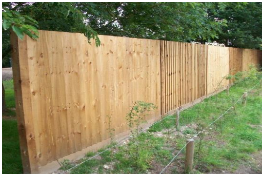
1.8m Close Boarded Timber Fencing to the Sides & Rear Boundaries
