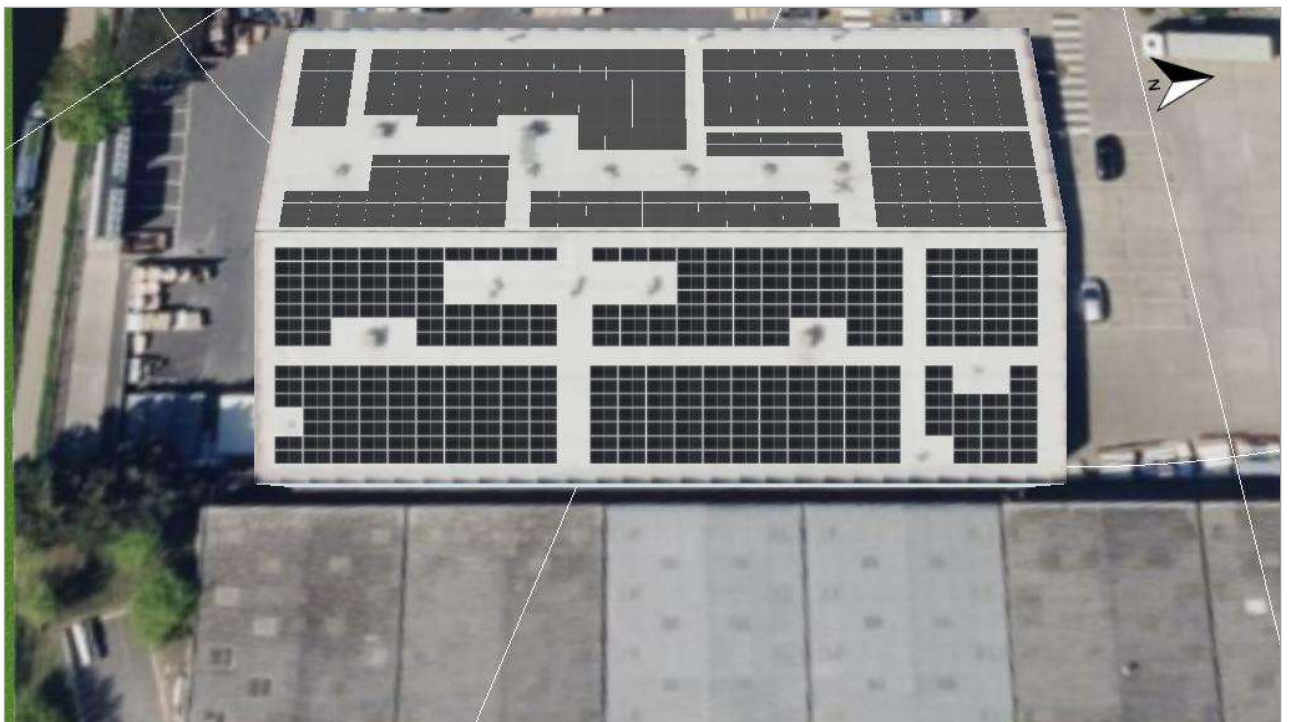
Figure: 1. Module Area - Building 01-Roof Area East
