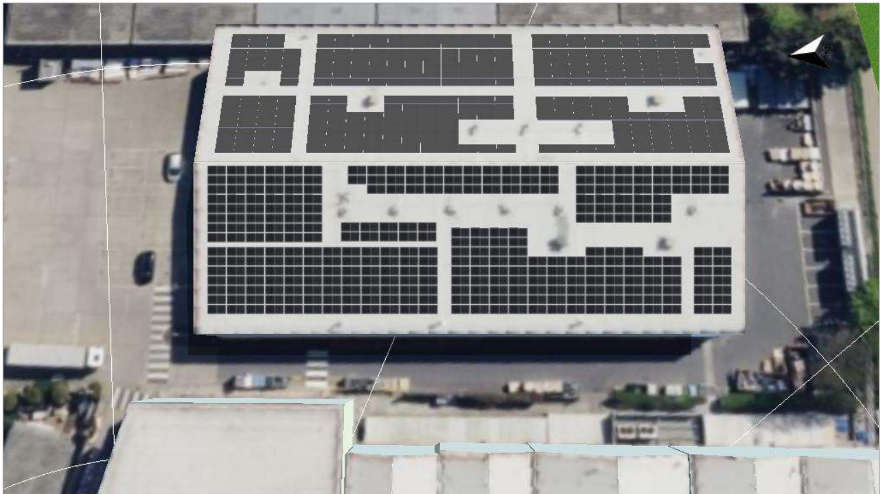
Figure: 2. Module Area - Building 01-Roof Area West
