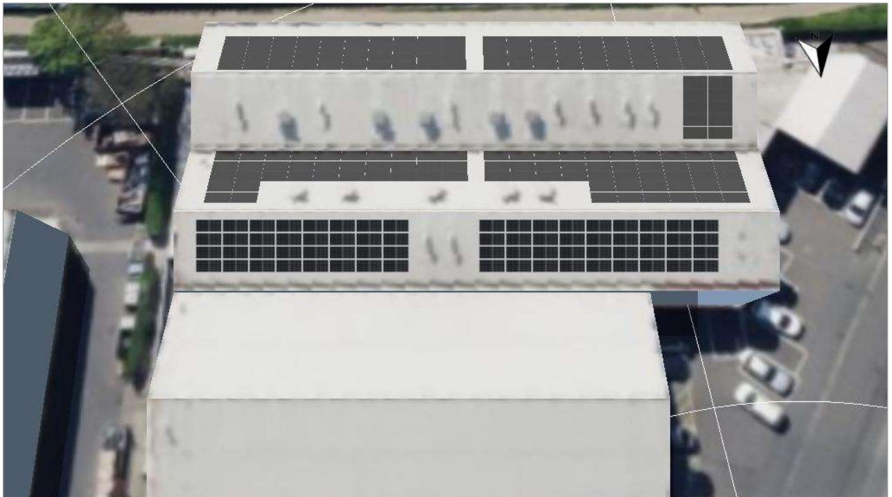
Figure: 4. Module Area - Building 05-Roof Area North
