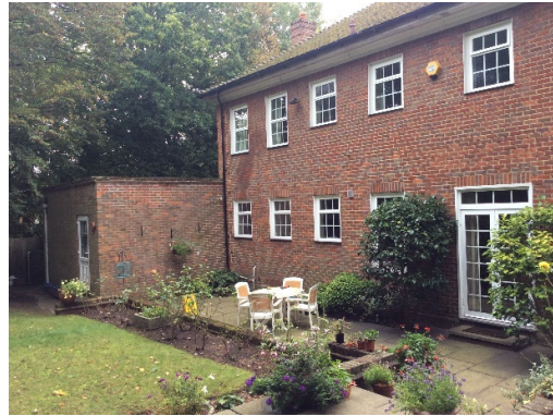
Rear View on Garage
