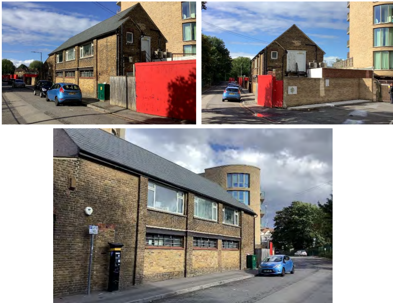
Figure 4: The study site showing the late-19 th century former printworks building (with later alterations).
