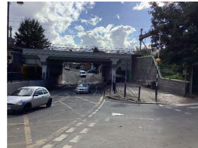
Figure 10: (top left): view along Tavistock Road showing large area of foliage-covered land which adjoins the railway; (top right): view from footbridge at West Drayton Station looking west; (bottom centre): view from corner of High Street and Tavistock Road looking south under railway bridge and showing raised embankment.
