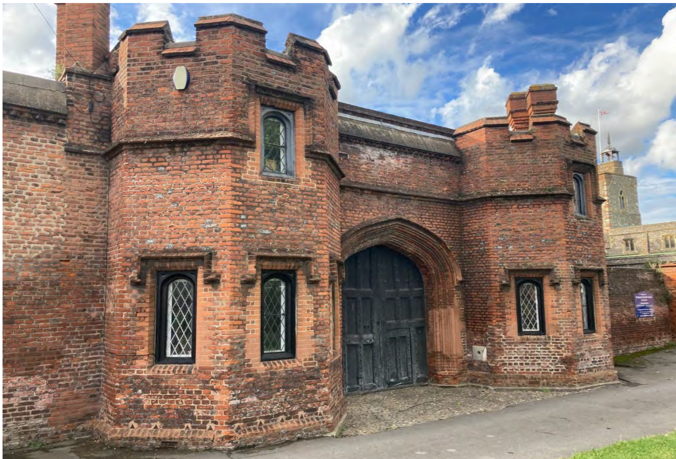
Figure 35: 16 th Century Gate House (Grade II*), formerly part of the Manor of West Drayton under the ownership of the Paget family, located at the top of Church Street, West Drayton.
