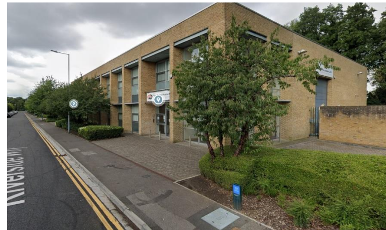
Fig 8. Existing Unit to the South West of the development site
