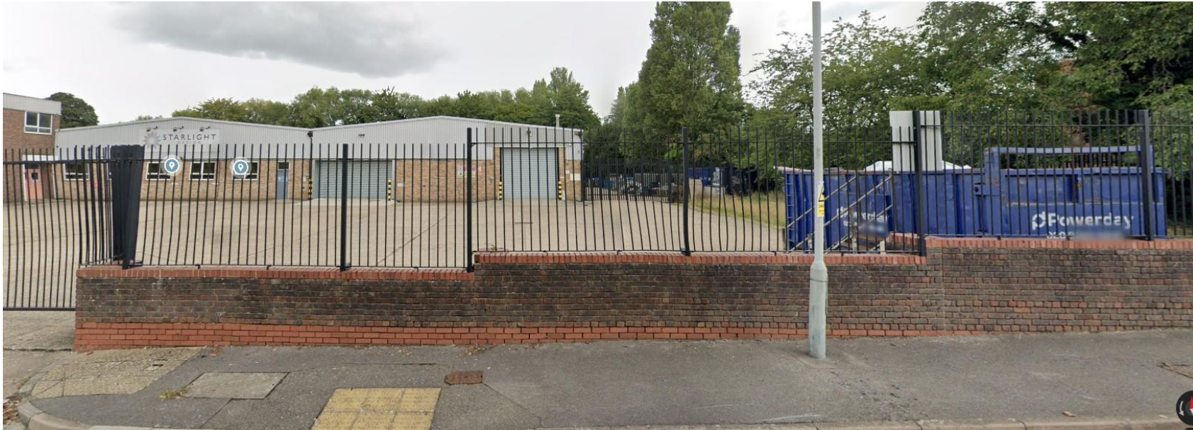
Fig 4. View of existing warehouse and external hardstandings.
