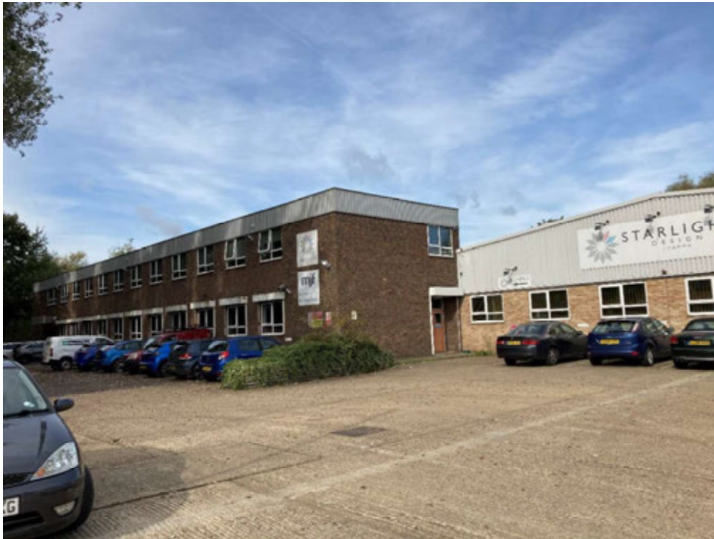
View of office building and attached warehouse (facing northwest)
