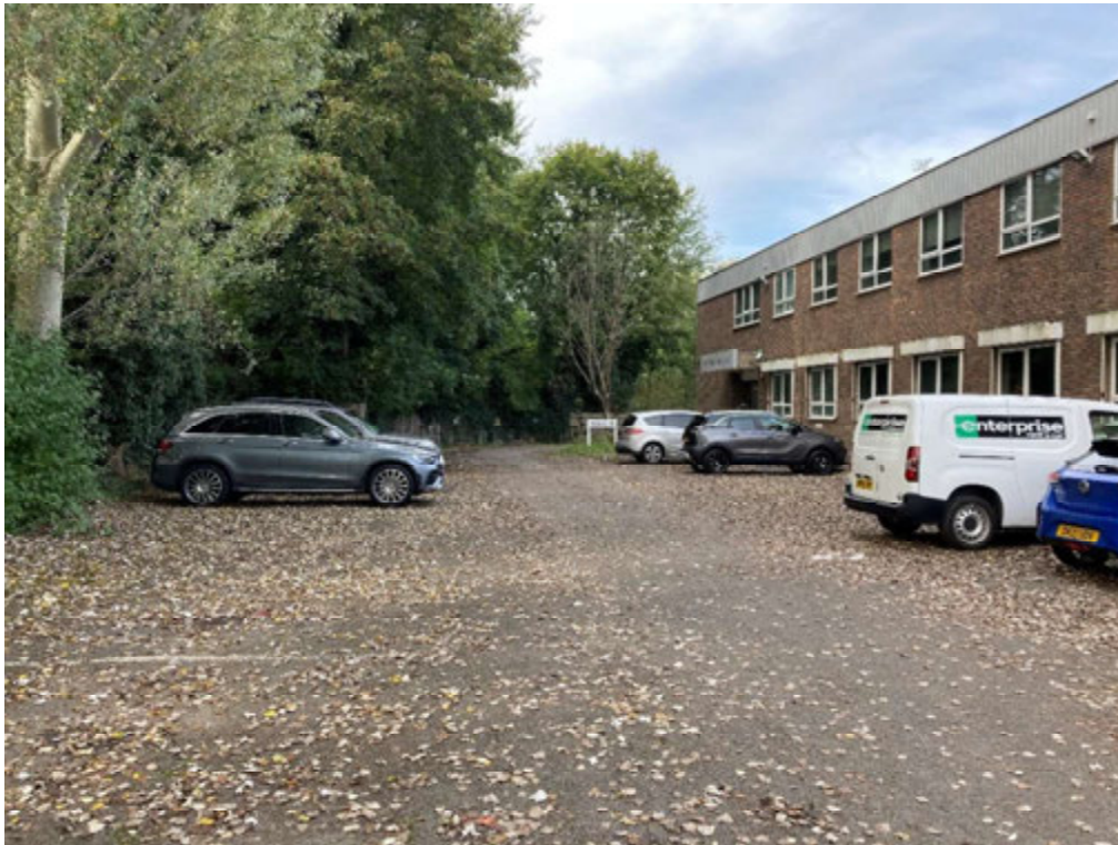
View of southern car park area (facing west)
