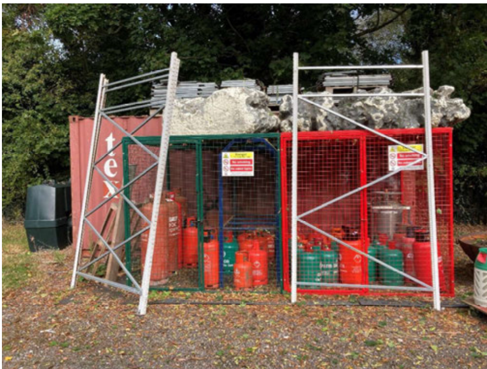
LPG storage cage and AST in the northern area of the Site (facing north)
