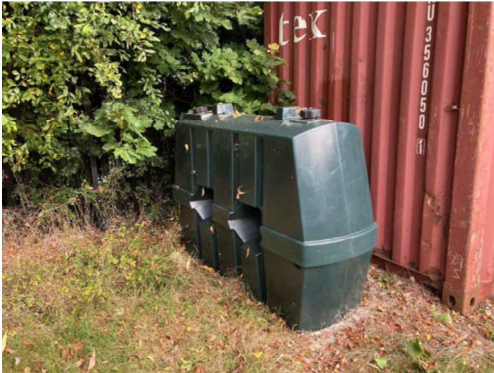
AST on the northern boundary of the Site
