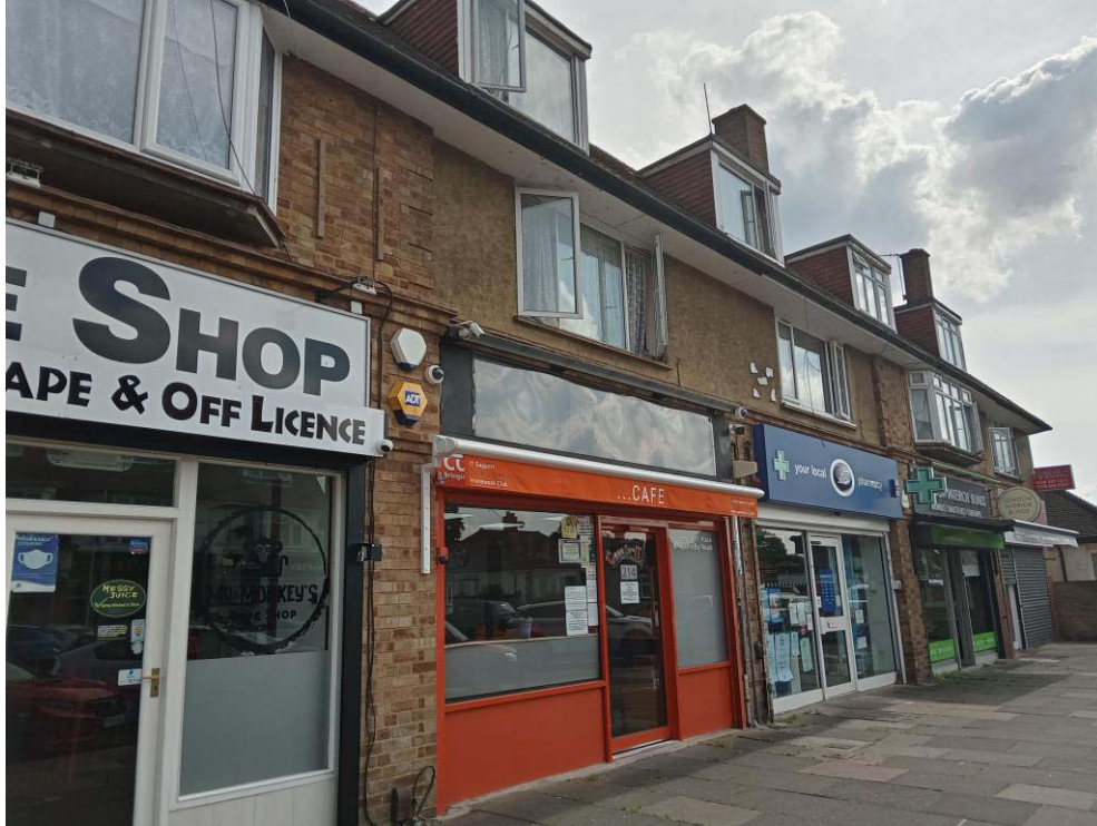
Photo 2: Pavement access directly outside site with parking bays.
