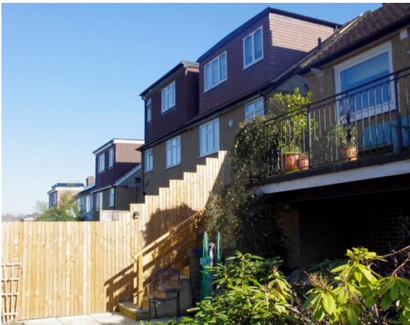
View 3 – Lower & ground levels of No. 72 from rear lower ground patio
