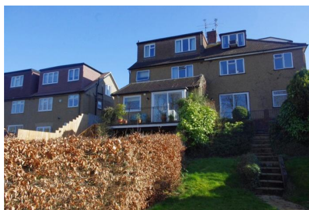
No. 74 to 66 Highland Road from rear garden
