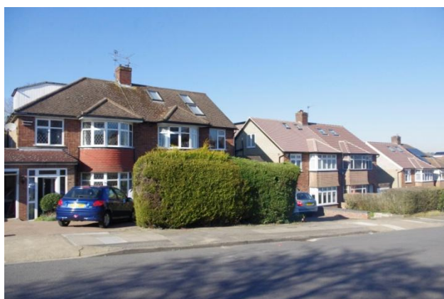
No. 74 to 62 Highland Road
