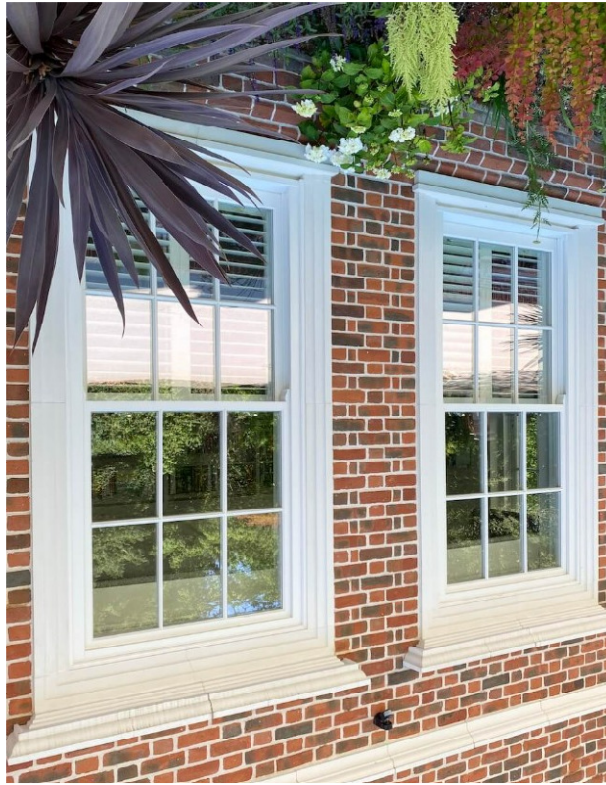
White timber sash windows with decorative beads
