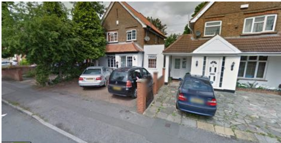
5.2 View looking North of adjacent property no. 76 Kingsway
