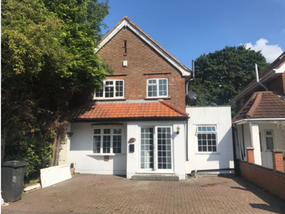
5.1 View looking North (Front) 78 Kingsway.
