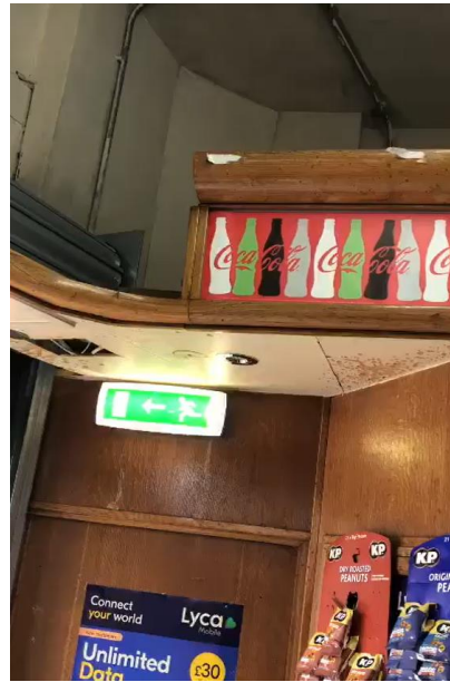
Figure 15 – Damaged timber coving detail to be removed
