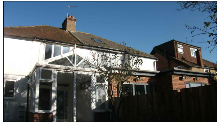
EXISTING REAR PICTURE SHOWING NUMBER 46 EXTENSION
