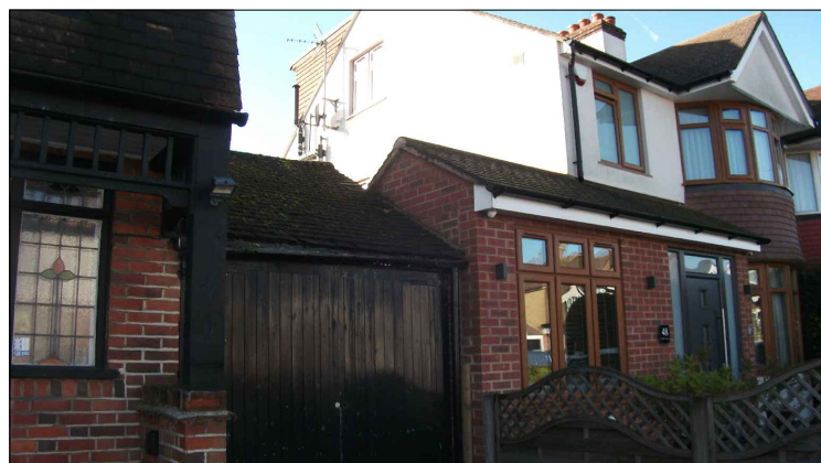
EXISTING FRONT PICTURE SHOWING GARAGE AND NUMBER 46 EXTENSION
