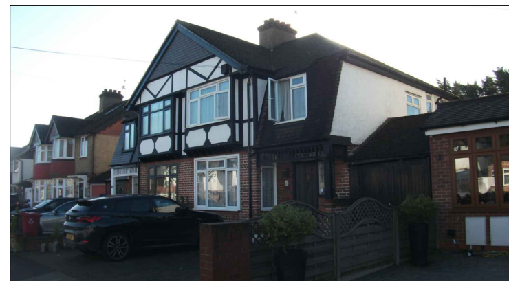
EXISTING FRONT PICTURE
