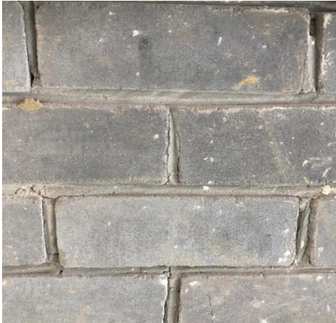
Original Bungalow brickwork and matched brickwork
