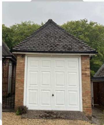
Building B2, southern elevation
