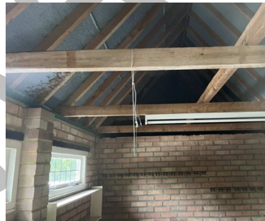
Building B2, interior, facing south
