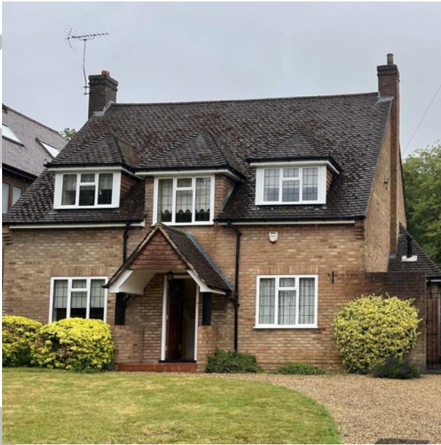
Building B1, southern elevation
