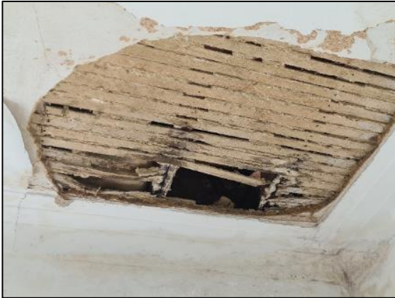
Photograph 15: Hole in ceiling into roof void.
