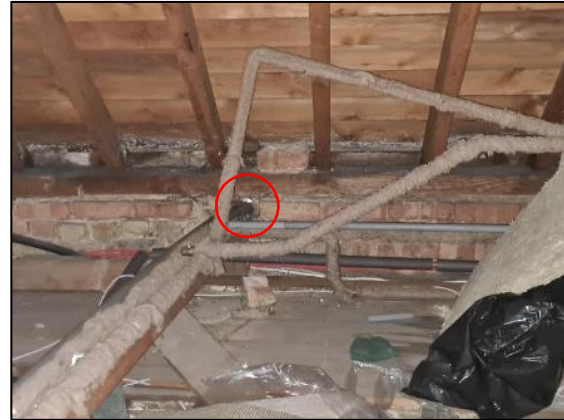
Photograph 16: Small gap around pipe.
