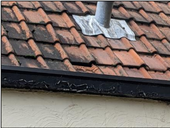
Photograph 11: Slipped tile on rear of the main building.
