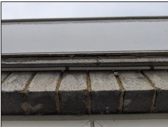
Photograph 13: Small gap under the boarding around the top of the extension.
