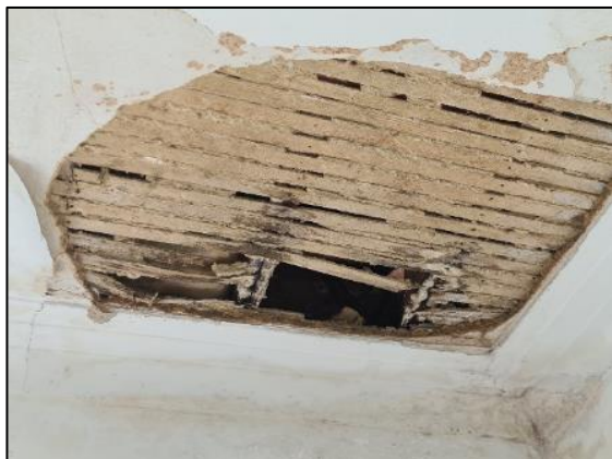
Photograph 15: Hole in ceiling into roof void.
