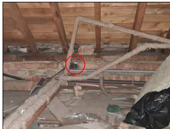
Photograph 16: Small gap around pipe.
