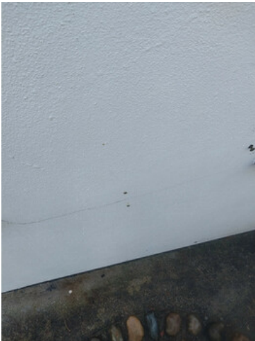
Ext front elevation between windows - Visit #4
