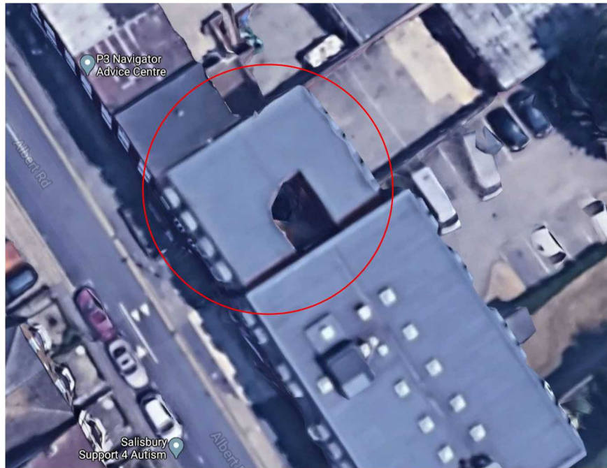
PHOTO 1: SHOWING REAR OF THE APPLICATION SITE
