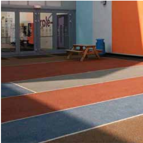
2 PAVING: Coloured tarmac surface (permeable) NTS Approximate area - 770 sq.m.
