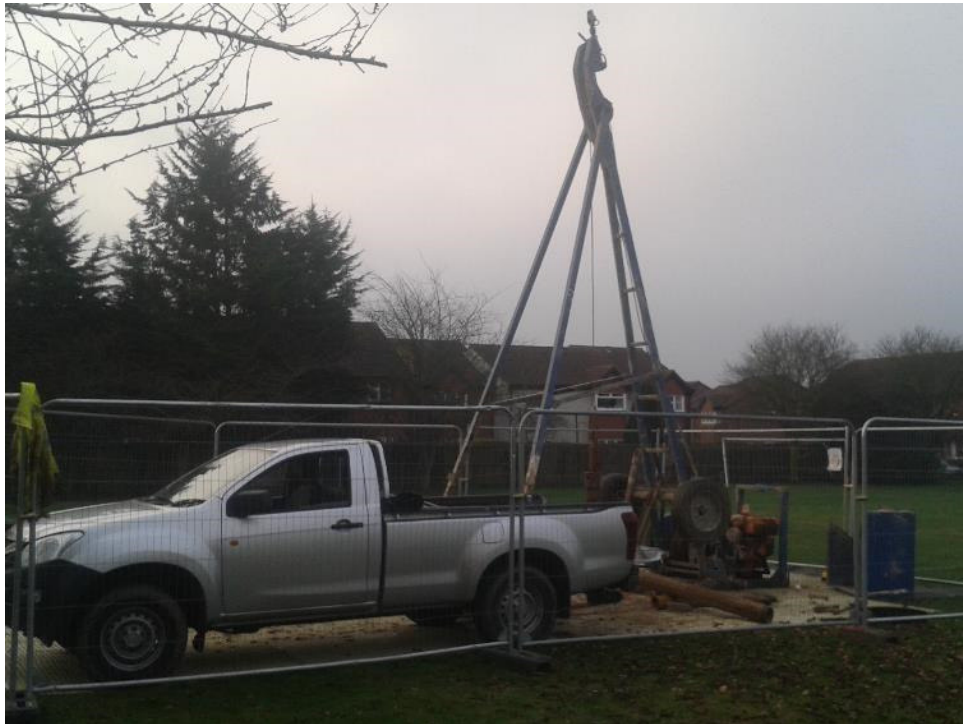
Photograph 5: View of rig setup at BH03
