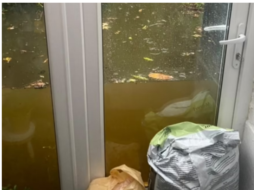
Figure 9: UPVC doors under flood conditions. These appear to offer reasonable flood resilience
