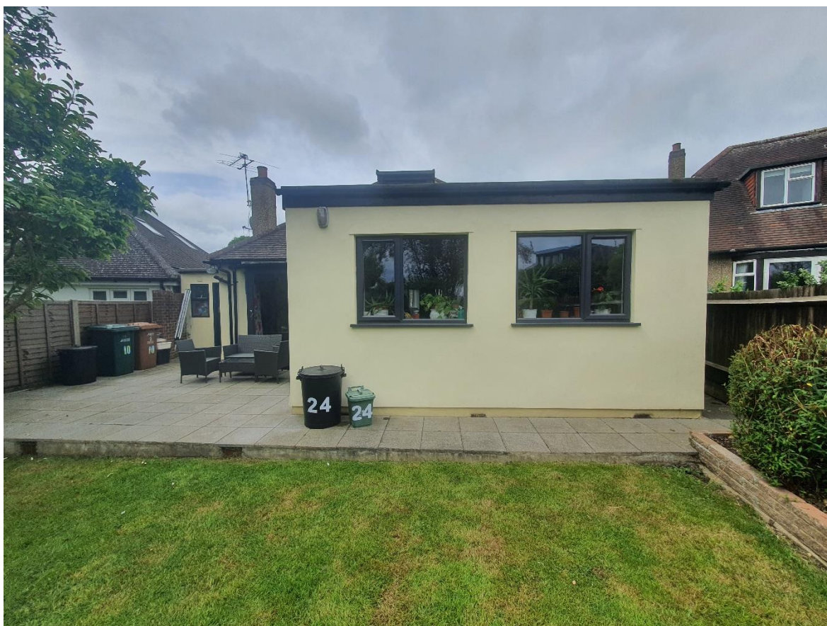
Rear of application property Including neighbour real elevations ( standing midway in garden )
